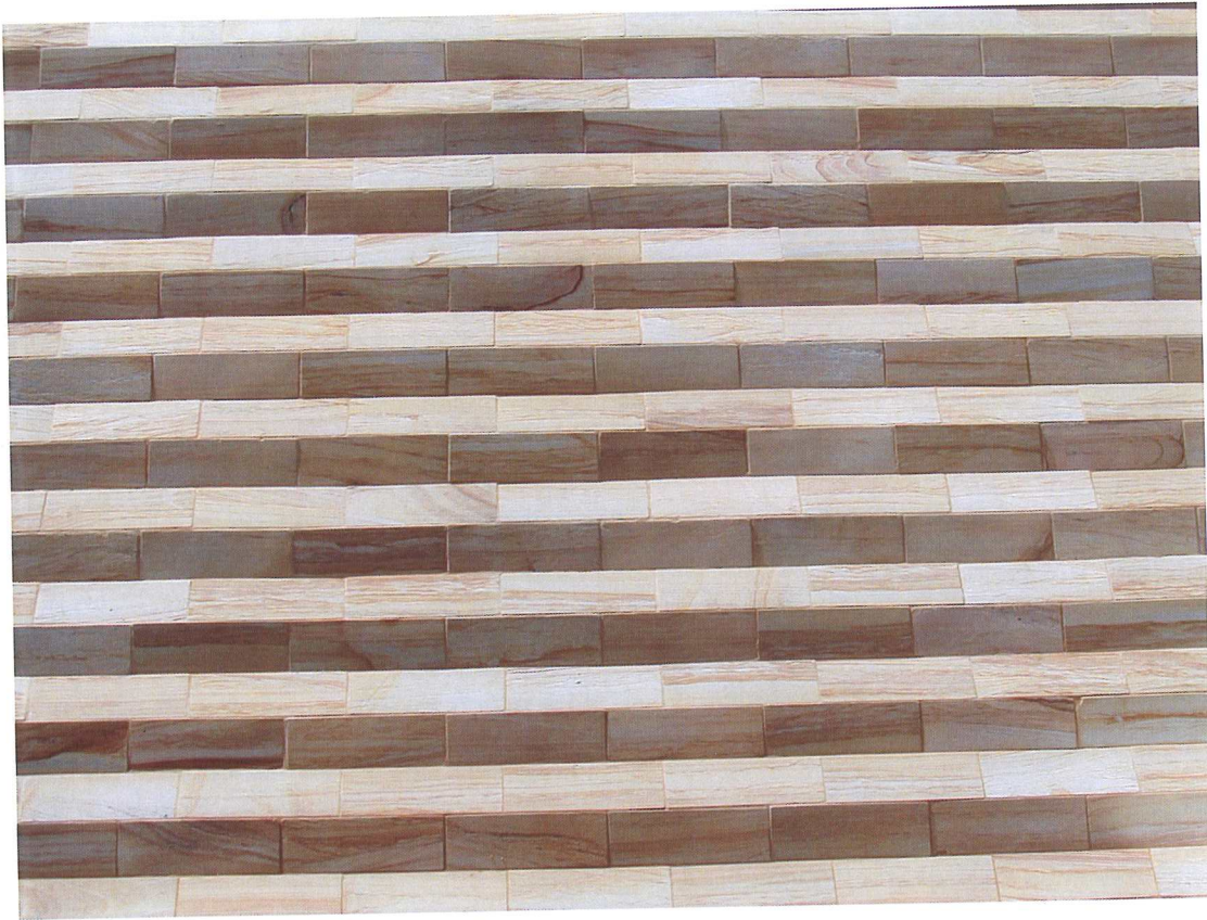
Fig. 3.1 Stone Wall Detail of House in Adelaide, (2002) Photo: Sam Ridgway
