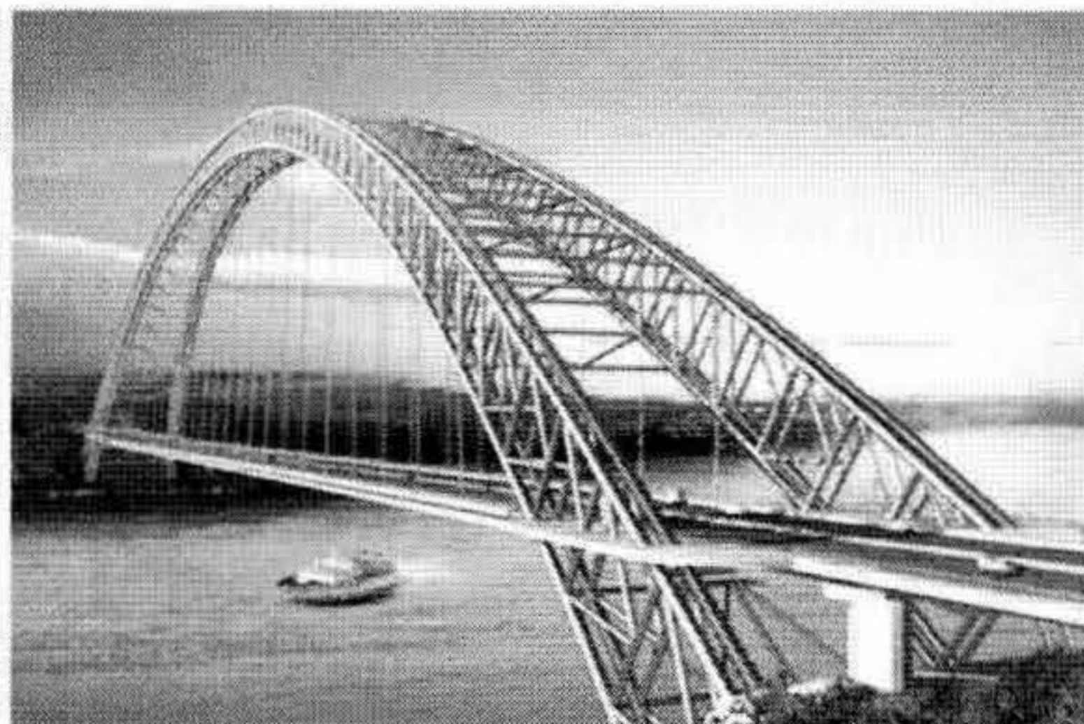
Figure 2-18 He River No. 1 Bridge
