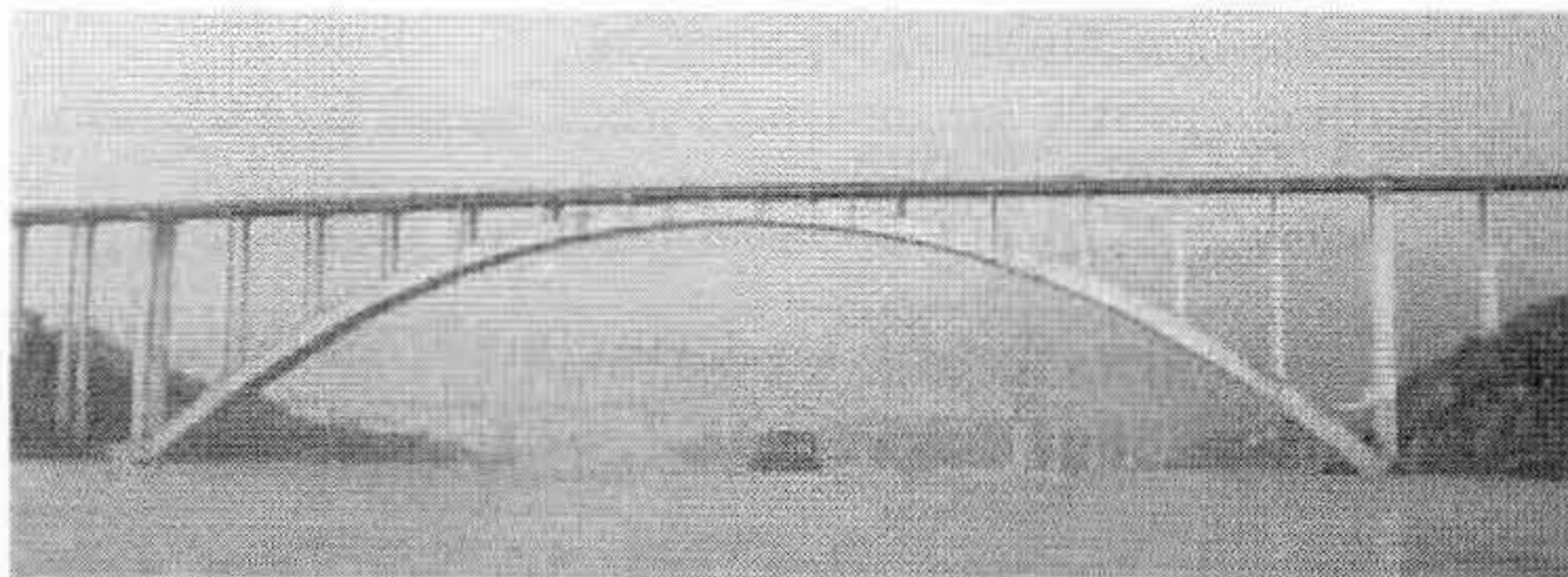
a) Whole Bridge
