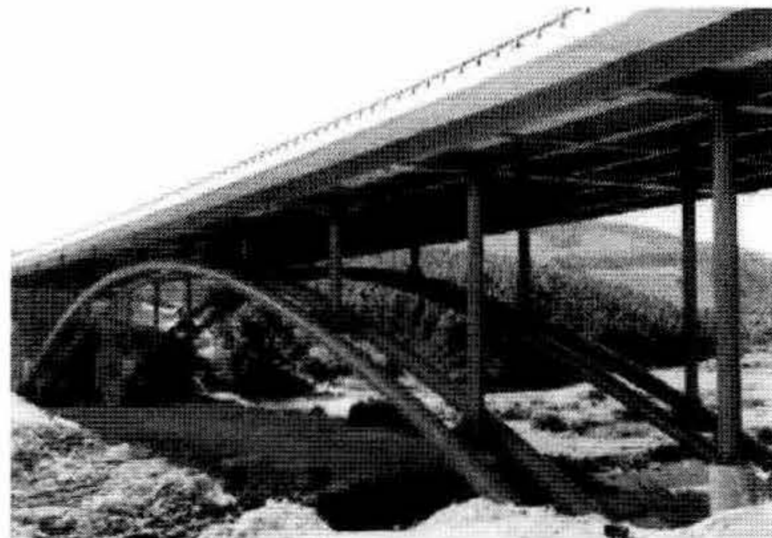
Figure 2-10 Arco del Escudo Bridge (Šavor & Bleiziffer 2008)
