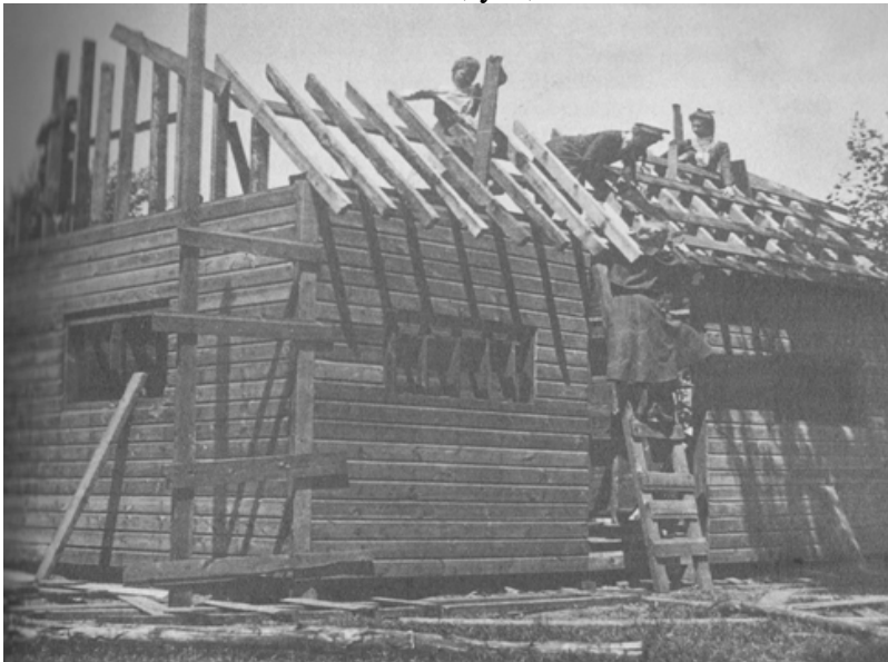
Fig 4. Tool shed being built by students. 24
