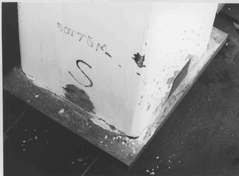
PLATE XXIV LOCAL COMPRESSION FAILURE AT ENDS
