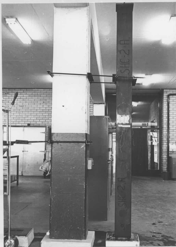
PLATE XXI HOLLOW SQUARE STEEL TUBE IN POSITION FOR CASTING OF CONCRETE
