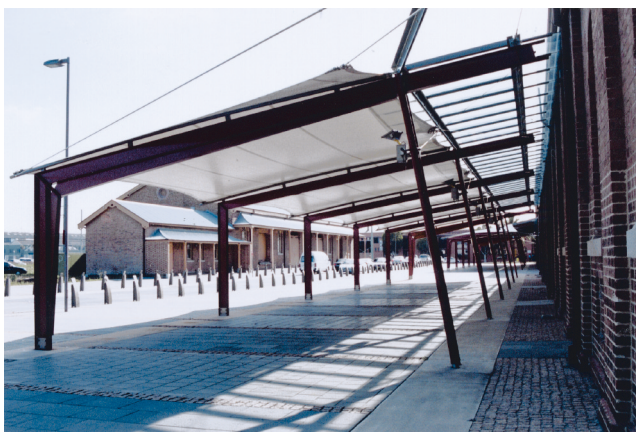
Illustration 4.37 Fabric awning, railway maintenance workshops
