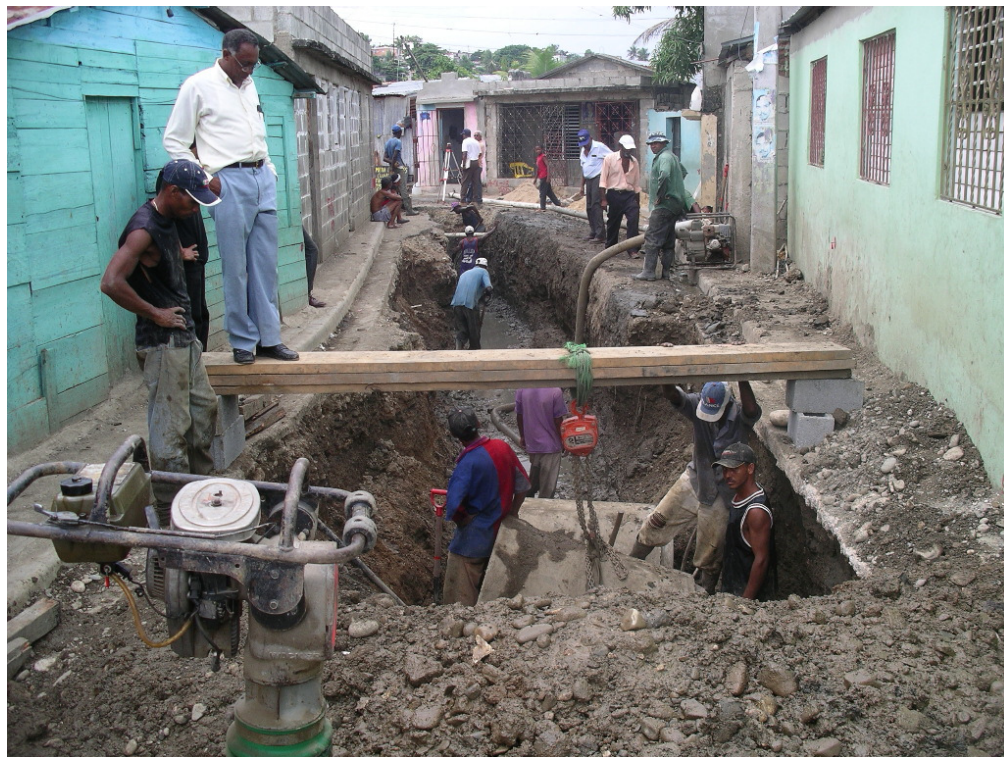
Figure 18. Installing stormwater drains in Calle 5, La Ciénaga.
