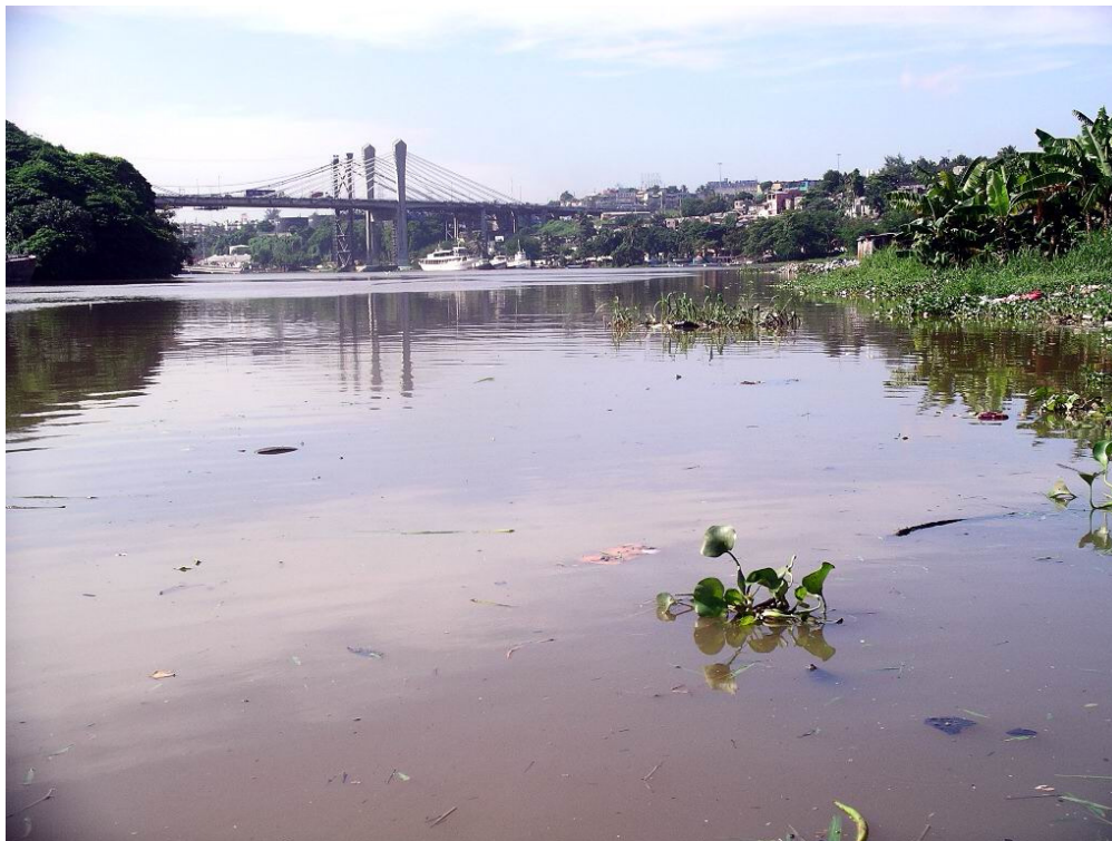
Figure 2. View of Puente Juan Bosch from the River Ozama next to La Ciénaga.
