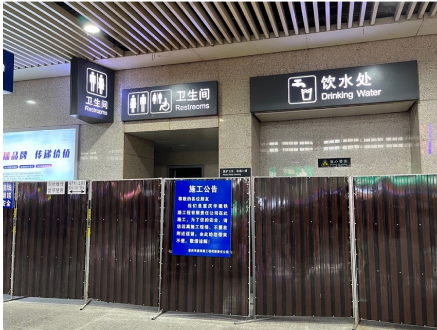
Figure 6. 14: An under-maintenance area
