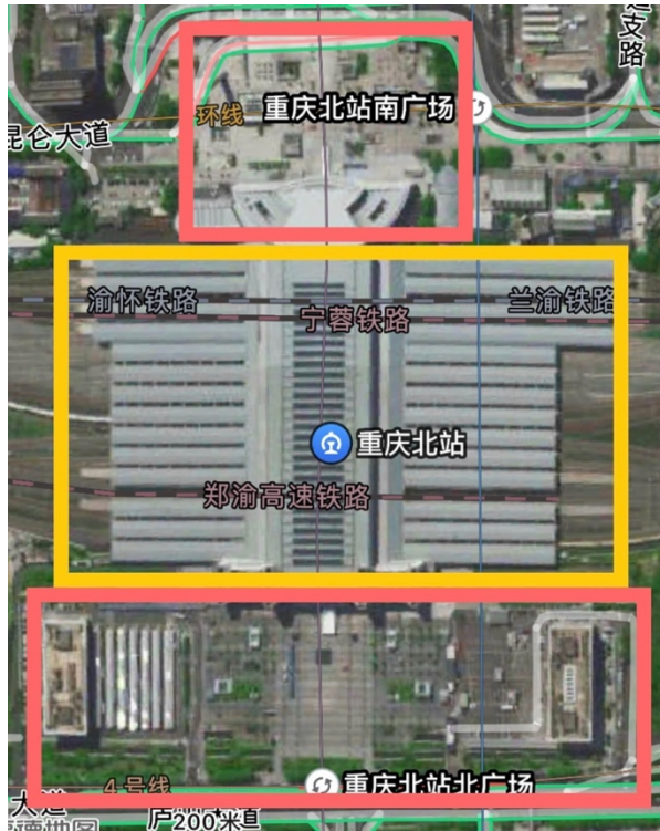
Figure 6. 2: Panoramic view of Chongqing North High-speed Railway Station
