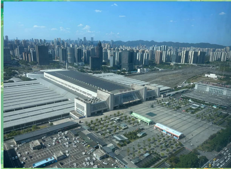
Figure 6. 4: Birdseye view of the north ground plaza 33
