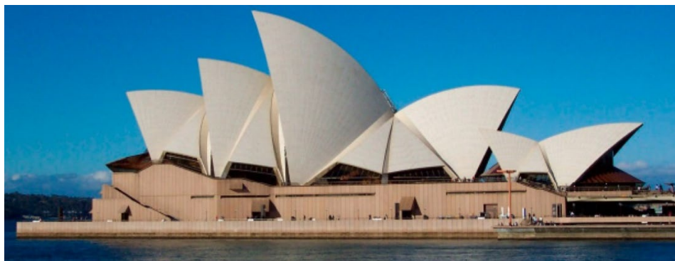
Figure 1.1 Over 1,400,000 tiles on the Sydney Opera House [14]
