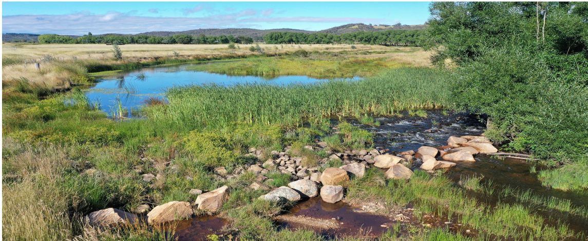
Figure 3: Leaky weir at 'Westview Farm' - a log sill (woody) weir built in 2019. The logs are hidden by a rocky baffle. This weir is considered by the Mulloon Institute as one of their most successful projects to date. Credit: Mulloon Institute, 2020.
