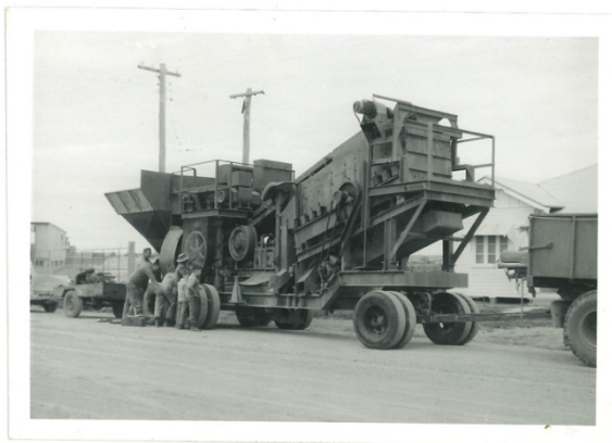
Figure 6. Jack Harman, North west concrete crushing plant used on the Narrabri to crush gravel (recto and verso), 2025, digital scan from archival record.
