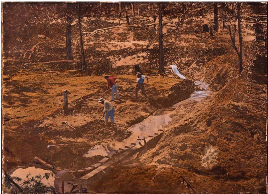
Figure 27. Richard Daintree, Alluvial Gold Mining, Creek Sluicing, 1864-1871, Albumen print, overpainted, mounted on textile support, on wooden stretcher, nails, 44.3 x 60.8 x 2.0cm
