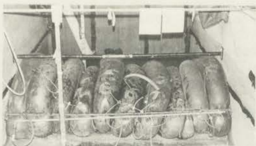
DIAGRAM 9.9 - INTERNAL HEAD 5 ft, U/S=0 NOTES: 1. A 1 INCH PVC HOSE WAS IN- SERTED TO ALLOW AIR TO ESCAPE FROM IN- SIDE THE TOROID. 2. THE WATER-INFLATED TUBES APPEAR TO BE IRREGULARLY INFLATED.
