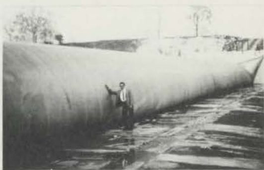
DIAGRAM 1.4 - A WATER INFLATED DAM ON LOWER COLORADO RIVER, BAY CITY, USA. (13 FT. HIGH BY 227 FT. LONG)
