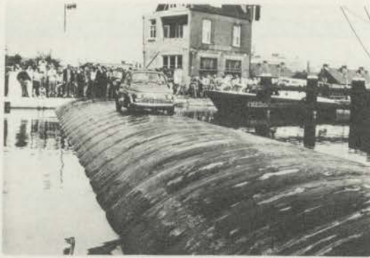
DIAGRAM 2.1 - BUIJZE -STEEL PANEL TYPE WATER INFLATED DAM, SHOWN HERE SUPPORT- ING LIGHT TRAFFIC. THE UPSTREAM AND DOWNSTREAM HEADS APPEAR ALMOST EQUAL.
