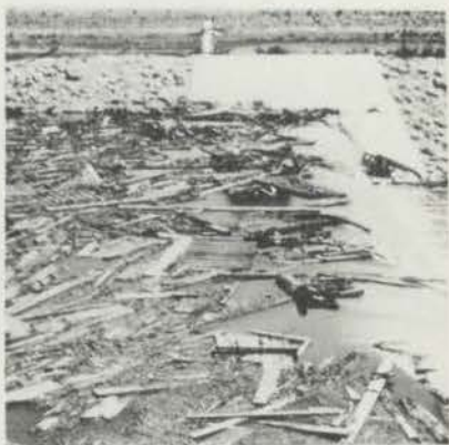
DIAGRAM 3.4 - THE USE OF AN INFLATABLE DAM AVOIDS THE POSSIBILITY OF DEBRIS JAMMING THE GATE. DURING FLOODS FABRIDAMS HAVE PASSED TREES & BOULDERS WITHOUT DAMAGE.
