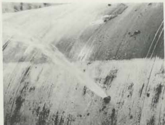
DIAGRAM 3.1 - PUNCTURED WATER-INFLATED DAM. RUPTURES OF THIS TYPE CAN EASILY BE PATCHED WHILST DAM REMAINS INFLATED.
