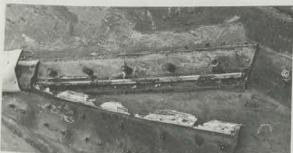
DIAGRAM 3.27 - SECTION OF TORN FABRIC ADJACENT TO WHERE FABRIC PULLOUT OCCURRED.
