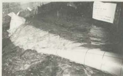
DIAGRAM 5.15 - ... AND TRAVELS TO AN END, RESULTING IN TOTAL COLLAPSE. FLOW 2.5 cusecs.
