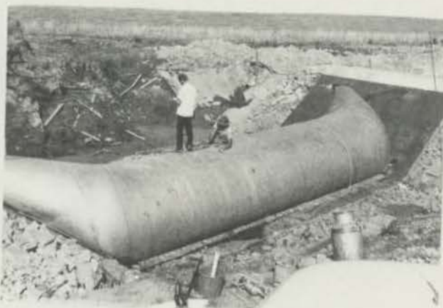
DIAGRAM 3.11 - FULLY INFLATED ALTHOUGH IT APPEARS TO BE DESIGNED FOR HIGHER UPSTREAM HEADS THAN DOWNSTREAM, THE DAM APPEARED TO FUNCTION SATISFACTORILY WHEN THIS SITUATION WAS REVERSED.
