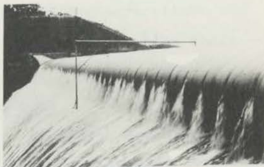
DIAGRAM 1.2 - INCREASING THE HEIGHT OF KOOMBOOLOOMBA DAM (TULLY FALLS, QUEENSLAND), FOR HYDROELECTRIC PURPOSES, BY THE INSTALLATION OF A 5' WATER INFLATED DAM. THIS DAM IS LOCATED ON TOP OF AN OGEE SPILLWAY.
