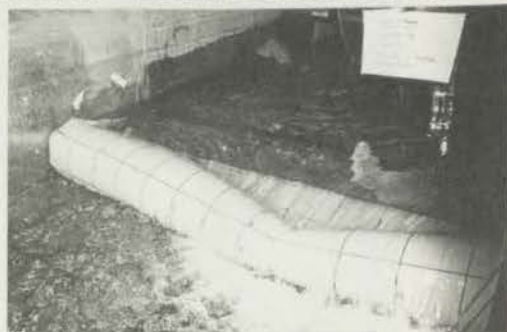
DIAGRAM 5.14 - A NOTCH IS BEGINNING TO DEVELOP WITH AN INCREASE IN FLOW AND REDUCTION IN AIR PRESSURE.
