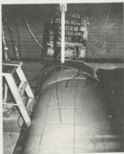
DIAGRAM 5.4 - A WATER-INFLATED DAM. APART FROM ONE OR TWO CREASES APPEARING NEAR THE ENDS, THE DAM BEHAVED UNIFORMLY.
