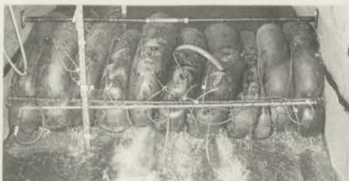
DIAGRAM 9.10 - CUSP LEAKAGE OCCURRING BETWEEN TUBES NEAR CENTRE AT U/S HEAD OF 2 FT.
