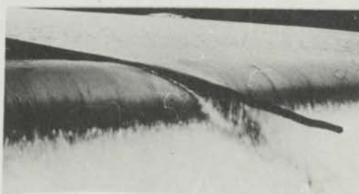
DIAGRAM 3.24 - A LOG PASSING OVER THE KOOMBOOLOOMBA FABRIDAM. THE OBJECT NUDDGES THE DAM THEN WORKS ITS WAY OVER IN A NOTCH FORMED BY ITS OWN WEIGHT.
