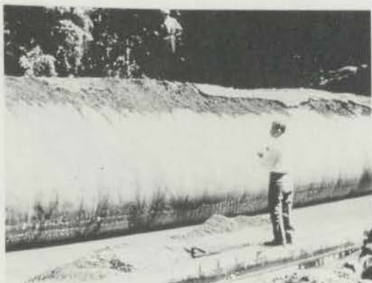
DIAGRAM 3.3 - THE POSSIBILITY OF A SILT LOAD SETTLING ON DEFLATED BAGS SHOULD BE CHECKED IN STRESS CALCULATIONS.
