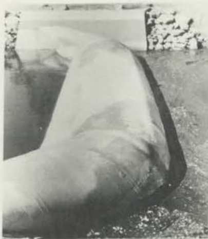
DIAGRAM 1.1 - A WATER INFLATED DAM USED AS A SALINITY BARRIER (ALUMY CK. NSW) TIDAL SALT WATER IS ON THE LEFT.
