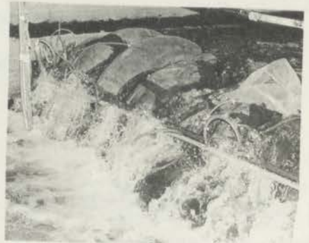
DIAGRAM 9.4 - WATER-INFLATED UNDER LOW INTERNAL HEAD, BEING OVERTOPPED.
