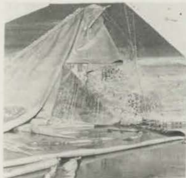
DIAGRAM 3.33 - THIS FAILURE STARTED IN THE LEFT-HAND DOWNSTREAM SIDE REGION UNDER A TEST LOAD. IT APPEARED TO RESULT FROM SIMILAR CAUSES TO THESE WHICH CAUSED THE 1969 FAILURE.
