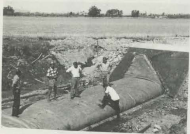
DIAGRAM 3.10 - PARTIAL INFLATION - CHECKING FOR LEAKS.
