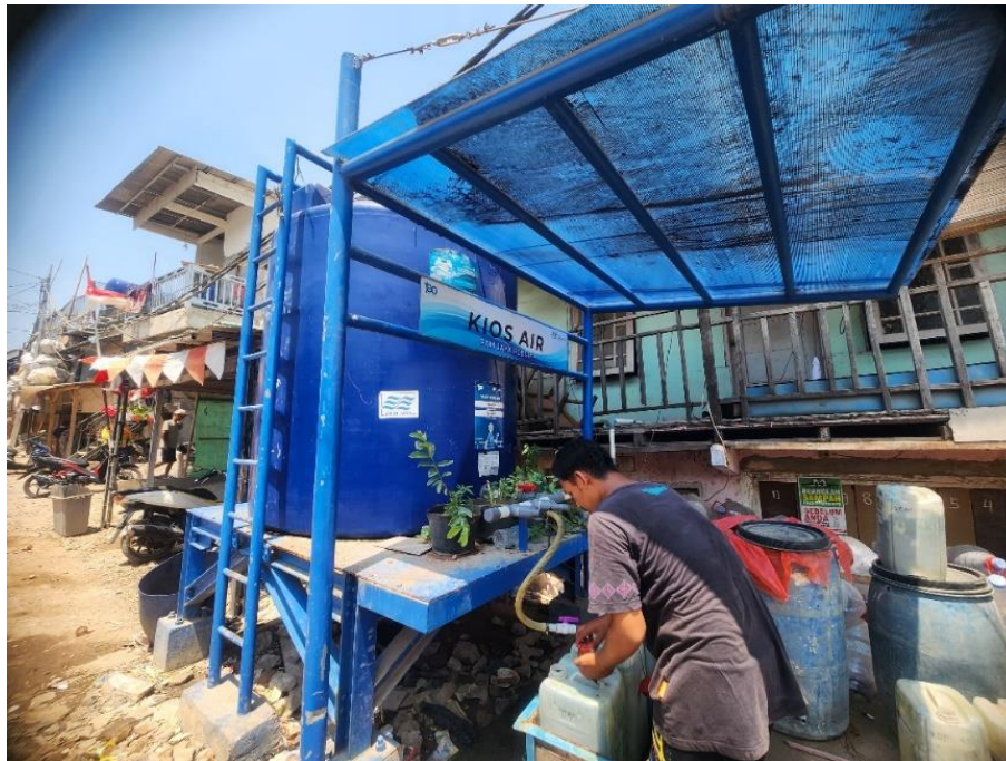
Figure 7.11 PAM Jaya's water kiosk
