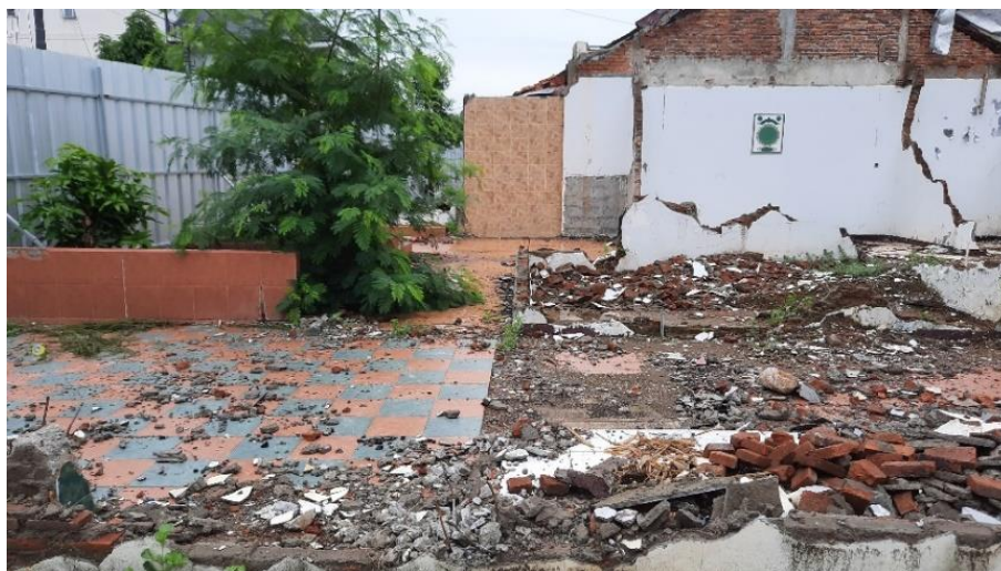
Figure 7.1 Rubbles in Kampung Poncol for WTP Bekasi
