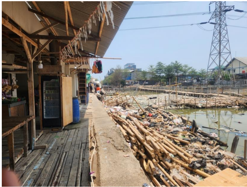
Figure 7.8 Houses sitting on the dike (above) and on marshland (below) in North Jakarta
