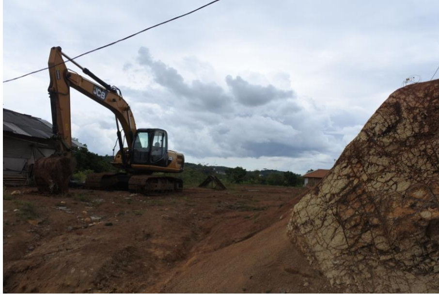
Figure 7.4 Flattening the ground for new settlement in Kampung Ciberang Baru
