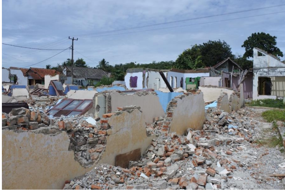
Figure 7.3 Rubble in Kampung Somang, Lebak, Banten.
