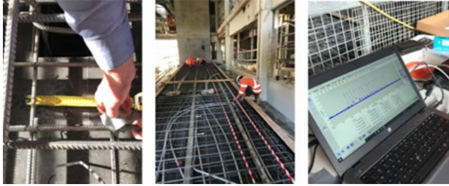
Figure 6.1 – Installation of FBG sensors during construction of the footbridge
