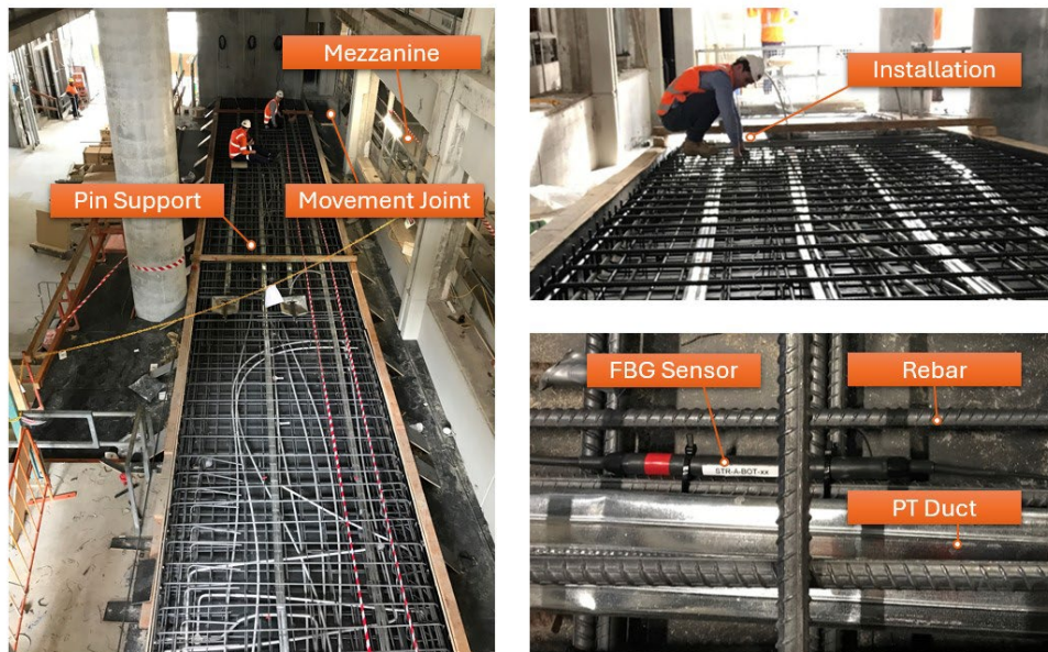
Figure 6.13 – Installation of Fibre Bragg grating sensors during construction
