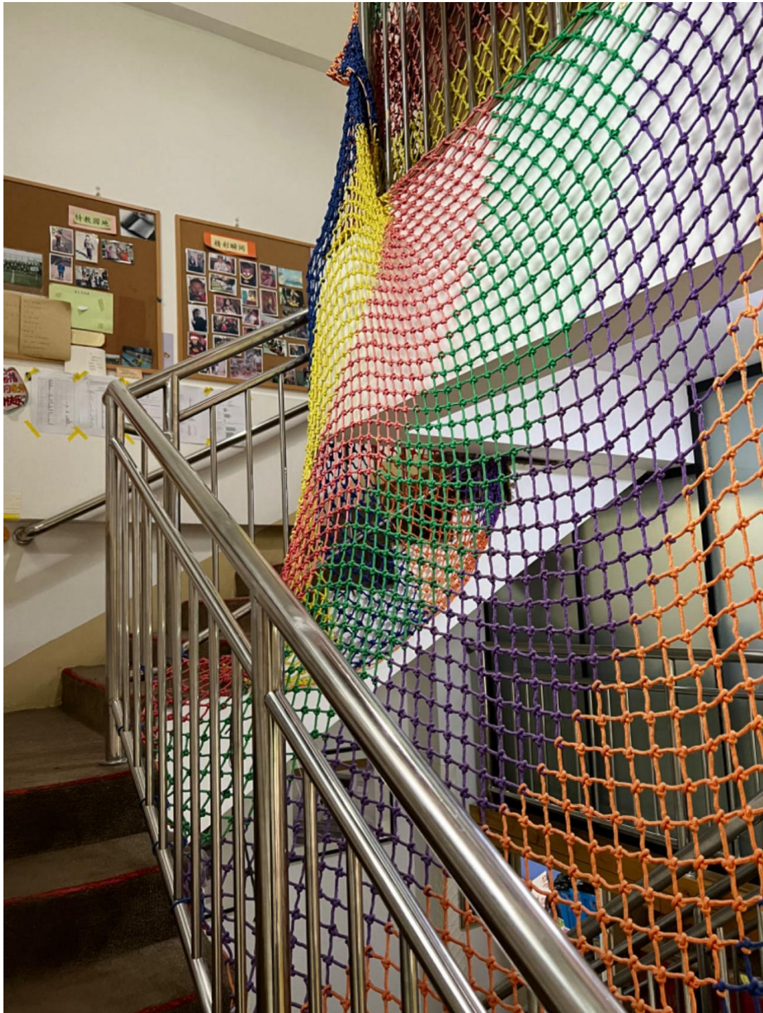
Figure 6.1. Coloured nylon netting hung between the first and first floor stairs.
