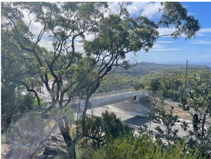
Figure 3: The Mona Vale Road pedestrian-style vegetated overpass following installation and planting and showing the duplicated Mona Vale Rd beneath.
