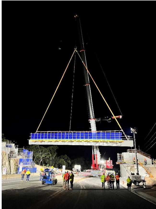
Figure 2: The Mona Vale Road pedestrian-style vegetated overpass being installed. Credit Jacqui Marlow.
