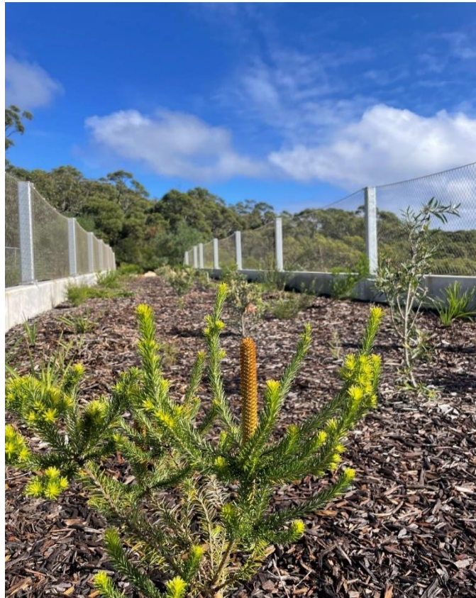
Figure 4: Mona Vale Road overpass, showing planted Banksia ericifolia and other shrubs to facilitate the movement of the eastern pygmy possum
