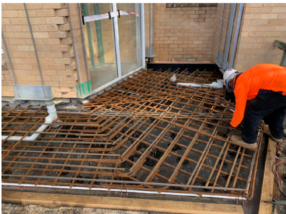
Figure 4-16 Rebuilding of new balconies; Source: MWA Architects
