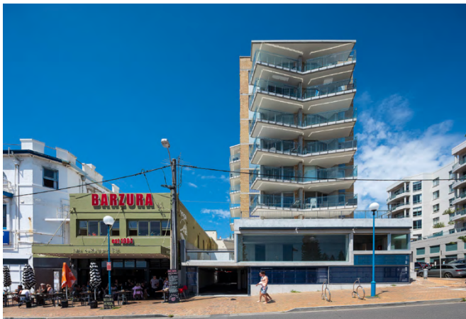
Figure 4-22 Coogee Waters post-renovation, North-facing facade; Source: Tom Ferguson
