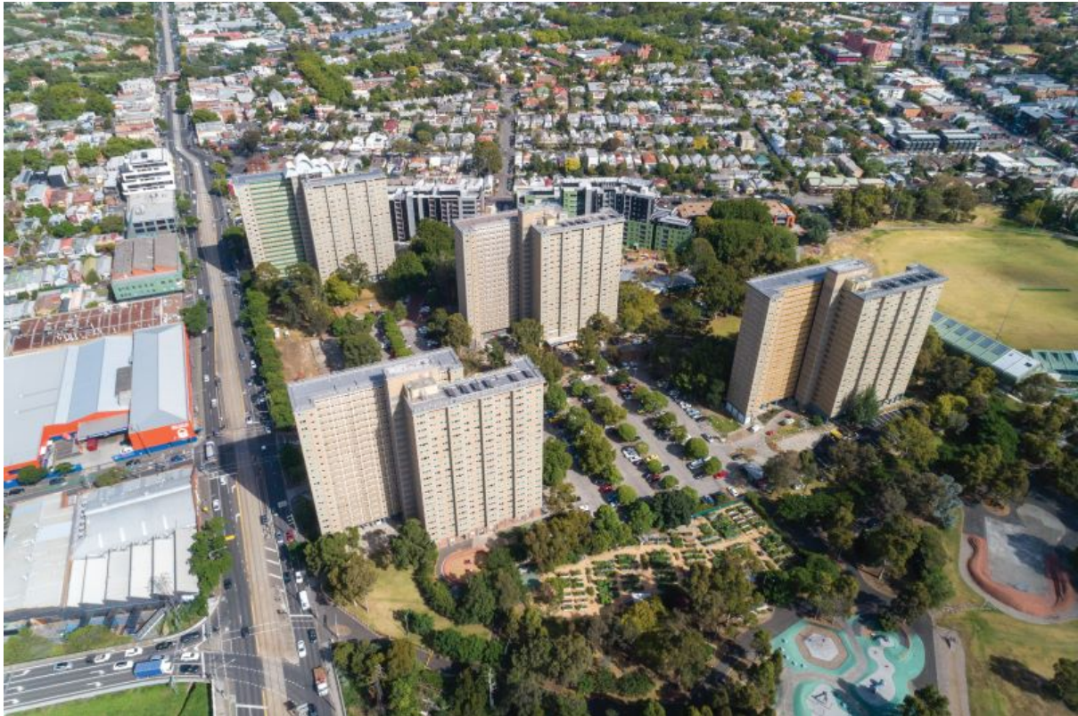
Figure 1-6 Example of a high rise pre-cast public housing towers in Melbourne built from 1962 to 1974 (Zeccola, n.d.)
