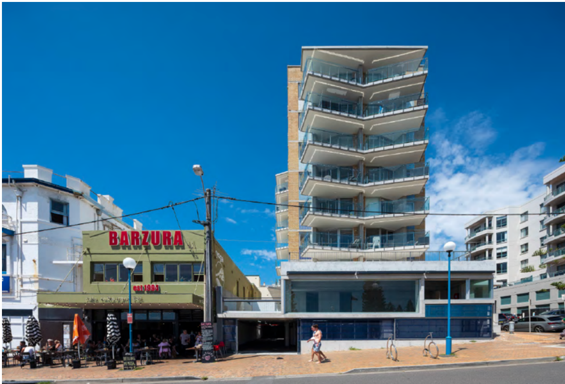
Figure 4-2 Coogee Waters post-renovation, North-facing facade; Source: Tom Ferguson
