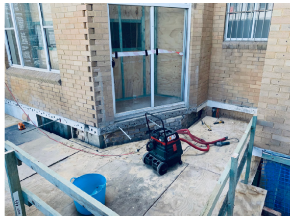
Figure 4-17 Rebuilding of new balconies; Source: MWA Architects
