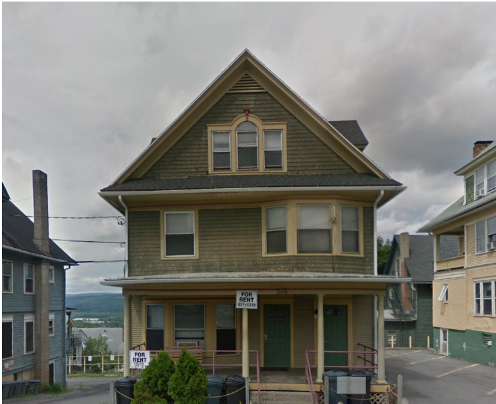
Figure 4-6 Catherine Commons, East-facing façade; Source: Google Street View, July 2018
