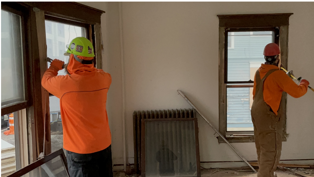
Figure 4-33 Preparing the building for deconstruction; Source: Joseph McGranahan (Circular Construction Lab, 2022a)
