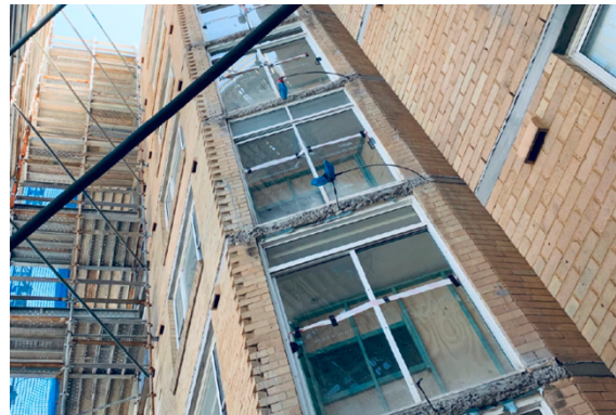
Figure 4-15 Previous balconies sawn off during construction stage; Source: MWA Architects
