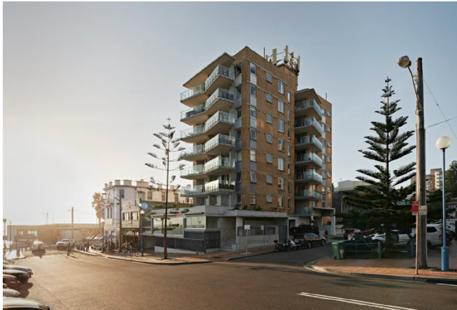
Figure 4-20 Coogee Waters post-renovation, North-West elevation; Source: Anthony Basheer
