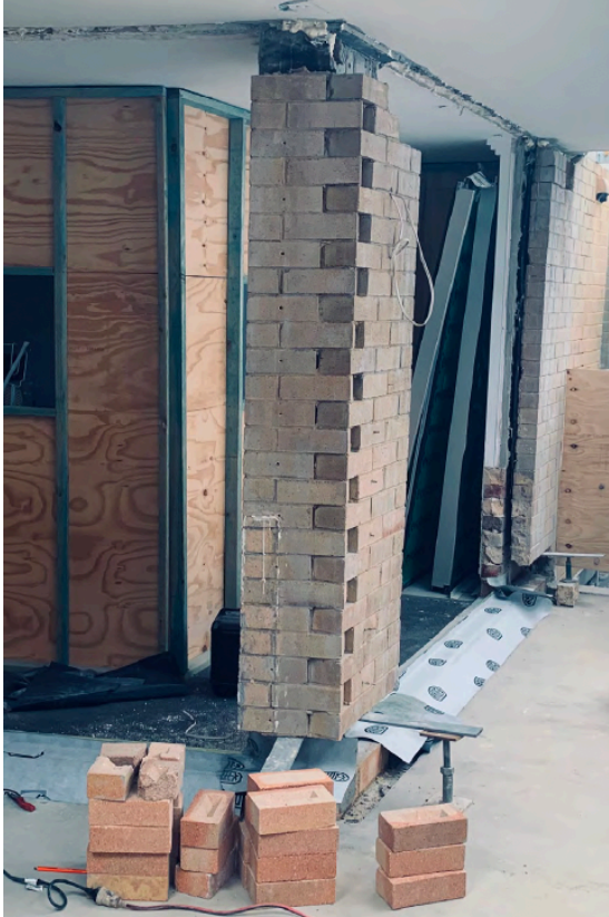
Figure 4-27 Brick ties being replaced with drill holes visible; Source: Project Architect
