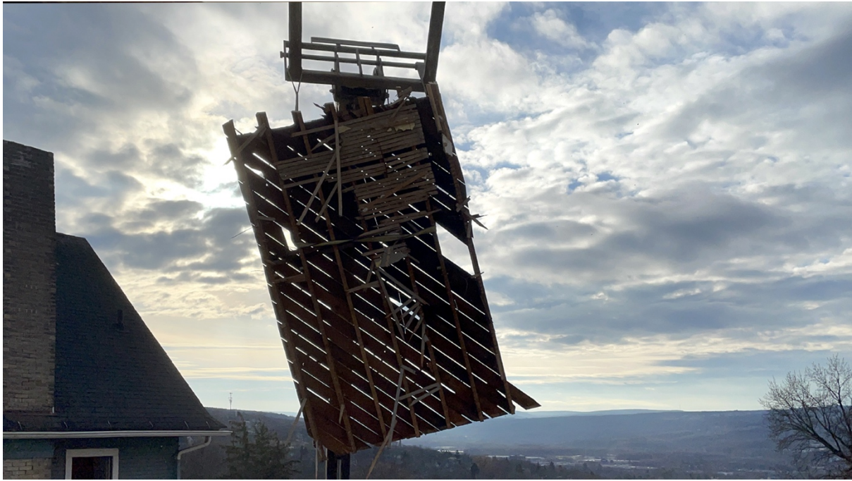
Figure 4-34 Deconstruction panel, Source: Felix Heisel (Circular Construction Lab, 2022a)
