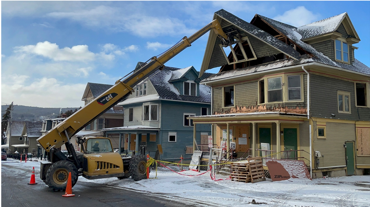
Figure 4-32 Deconstruction in Progress; Source: Felix Heisel (Circular Construction Lab, 2022a)
