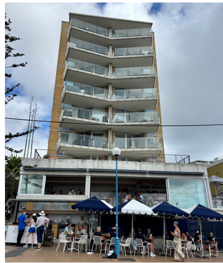
Figure 4-26 Coogee Waters post renovation, North-facing facade and cafe/restaurant in operation showing activated streetscape, Source: Author
