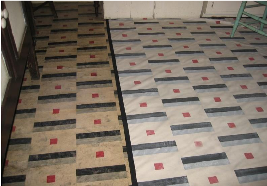
Figure 31. Meroogal Kitchen with protective transparent covering over original congoletum. Photograph taken by Suzanne Bravery, 2010, private collection.
