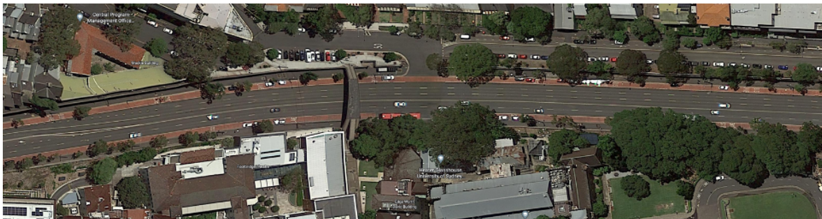
FIGURE 2.1: Peak hour only bus-taxi lane on Parramatta Road in Sydney, Australia. The lane is painted red and heavily used by buses. Bus-taxi lanes are commonly located on major bus corridors in Sydney. Source: Google Earth
