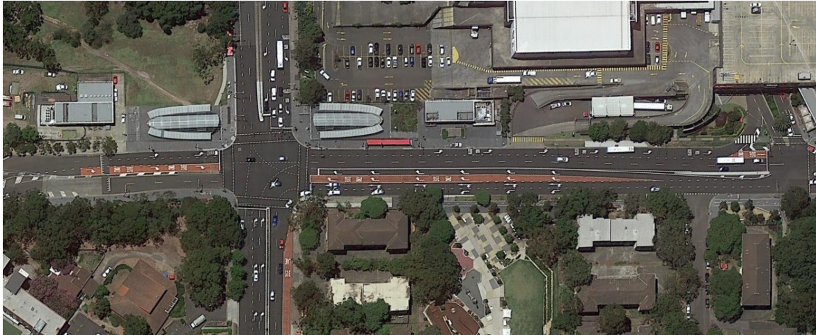
FIGURE 2.3: Cross-traffic turn queue jump located near Macquarie University in Sydney, Australia. The cross-traffic turn queue jump lane is positioned on the right side (east side) of the intersection. Large road surface is required to facilitate the cross-traffic turn queue jump lane. Source: Google Earth
