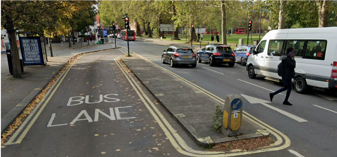
FIGURE 2.4: Bus pre-signal in Shepherd's Bush, London. Before the far side main signal turns green, general traffics are required to stop at the nearside pre-signal in order to allow buses on the bus lane to advance and skip the traffic queue at the intersection. The pre-signal reduces bus delay and allow easy access to right turn (cross-traffic turn) lane for buses at signalized intersection. Source: Google Earth Street View
