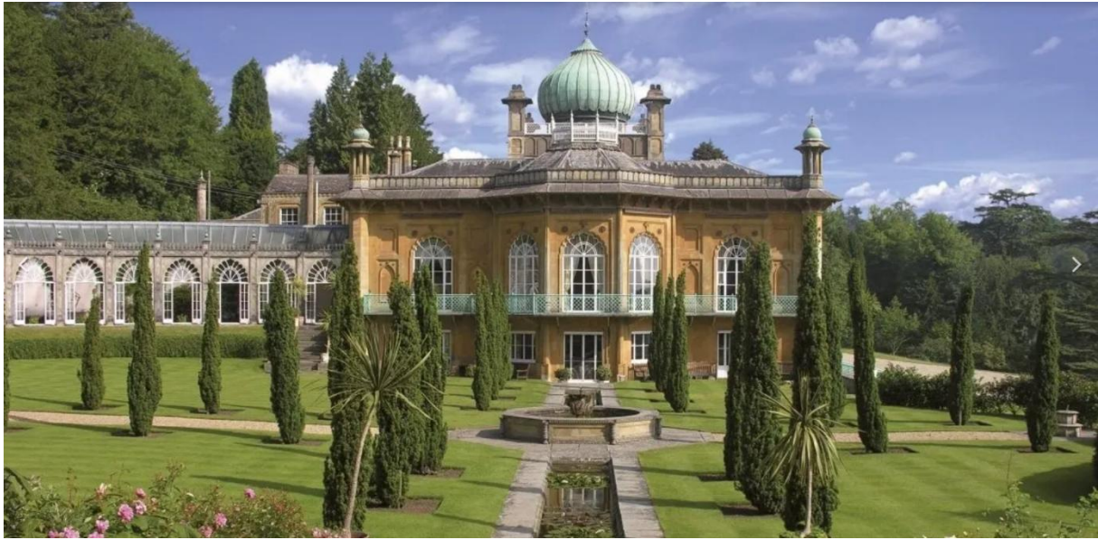
Figure 6. The Sezincote House in Gloucestershire 40
