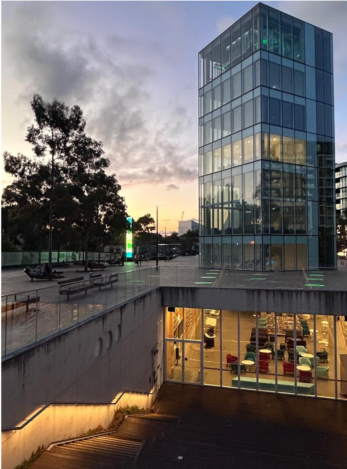
Figure 71 The amphitheatre connects the library and the open space, Green Square Plaza, January 2024.
