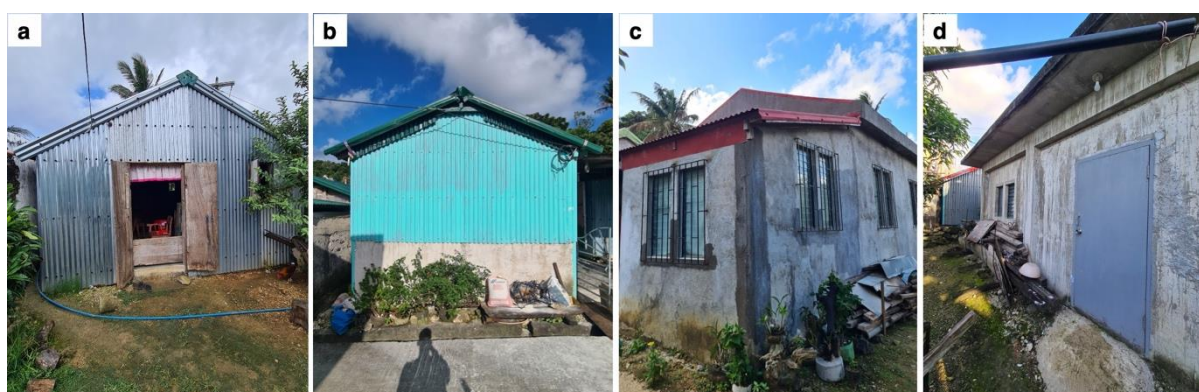
Figure 5.1. Predominant housing typologies in Itbayat, Batanes, Philippines. (a) A lightweight typology that can either have timber posts and beams (LWA) or steel posts and timber beams (LWB). (b) A semi-concrete typology that can either have steel posts and timber beams (SCA) or RC posts and timber beams (SCB). (c) An RC typology with lightweight roof (RCA). (d) An RC typology with RC slab roof (RCB).
