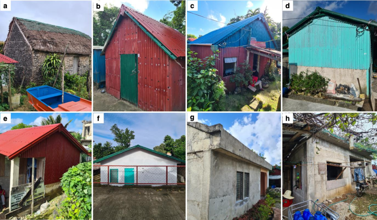
Figure 3.2. The surveyed housing typologies in Itbayat. (a) Unreinforced masonry (URM). (b) Lightweight with wooden posts (LW-A). (c) Lightweight with steel posts (LW-B). (d) Semi-concrete with steel posts (SC-A). (e) Semi-concrete with RC posts (SC-B). (f) RC structure with lightweight roofing (RC-A) where in some instances, inside gutters are common to conceal the edges of roofing sheets as shown in (g) . (h) RC structure with RC slab roofing (RC-B).
