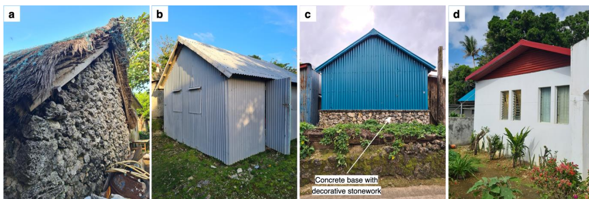
Figure 4.3. Emergent housing outputs. (a) Archetype of stone-and-lime vernacular house. Post-earthquake, the vernacular houses were damaged and were replaced with (b) lightweight, (c) semi-concrete, and (d) reinforced concrete typologies.
