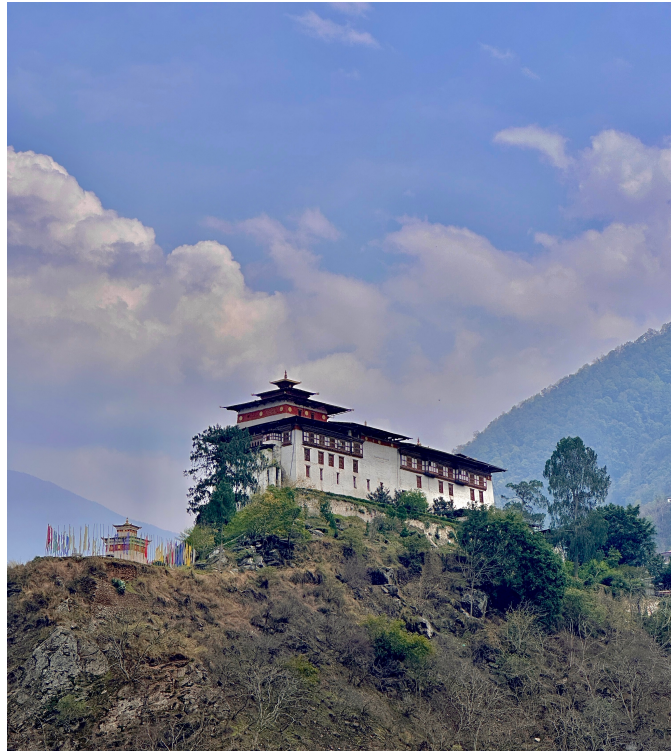
Image 1: Lhuentse Dzong- Fortress in the District of Lhuentse (Dzongs serve as the Headquarters of the District as well as the home to the monk body)
