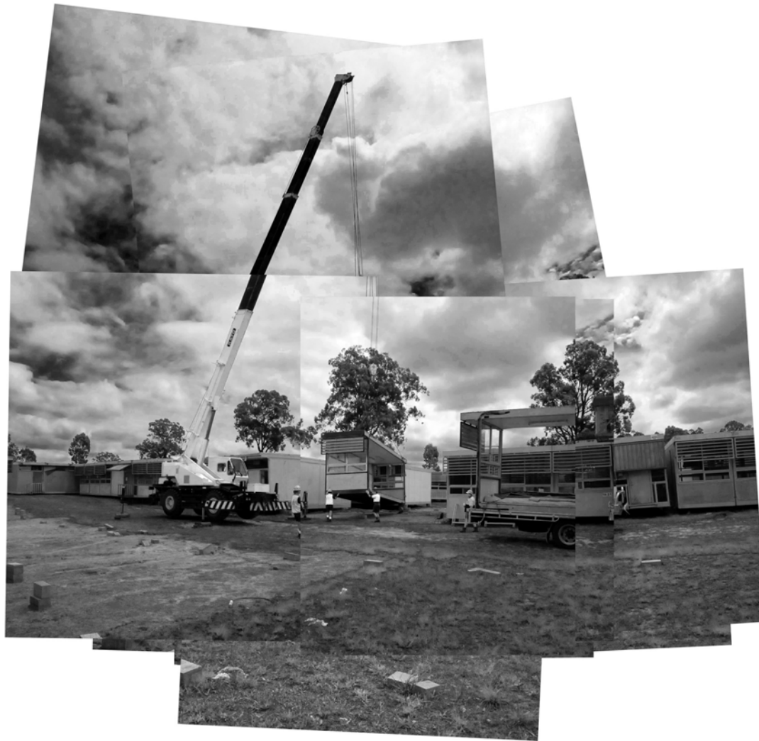
Figure 3.1: The movement of a Mk 1 Demountable Classroom during refurbishment in Cessnock. (The Author)
