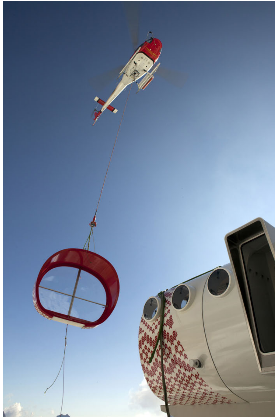
Figure 3.2: Construction of Refuge Gervasutti, Mont Blanc Massif, Italy A high performance prefabricated structure assembled at 2,500m above sea level cantilevered off the edge of a cliff above a glacier. It is designed to create thermally acceptable conditions inside in an environment that experiences extremes of hot and cold. IMAGE: Open Buildings, LEAPfactory Copyright: Francesco Mattuzzi
