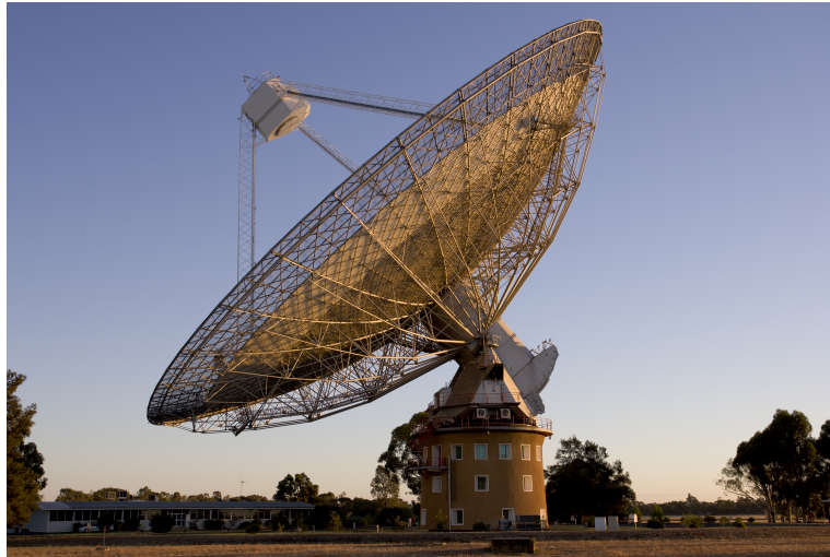
FIGURE 1.4. Murriyang, the 64 m radio telescope at the Parkes Observatory is an example of a single-dish telescope with a paraboloid reflector and receiver at the focus. Photo © Shaun Amy
