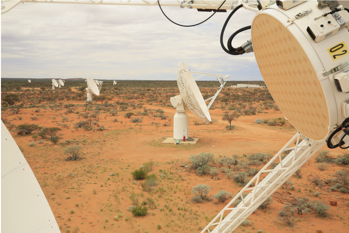
FIGURE 4.1. 12 m ASKAP antennas with PAFs at their foci at Inyarrimanha Ilgari Bundara, the CSIRO Murchison Radio-astronomy Observatory. Credit: CSIRO
