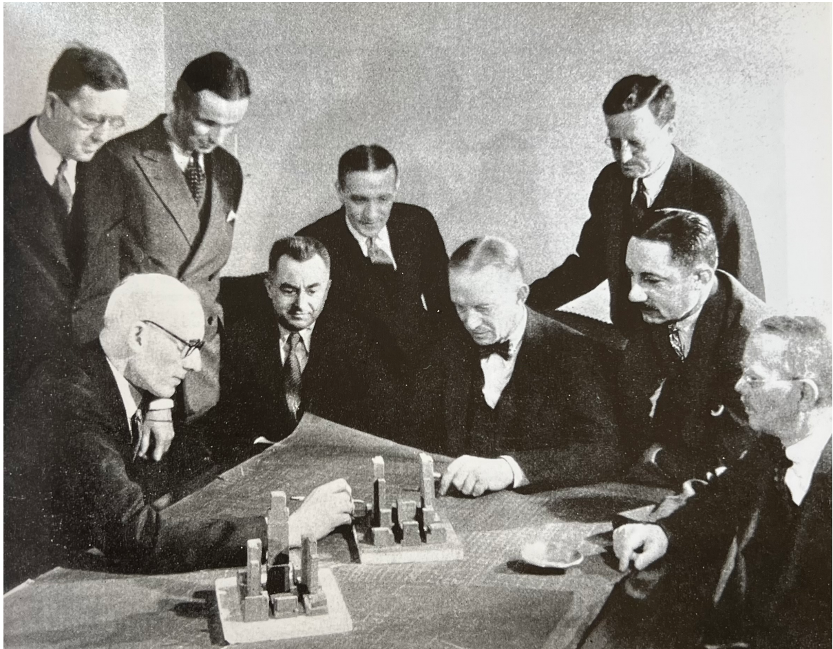
Figure 1.1 – Architecture by committee. This image shows Rockefeller Center's architects and developers using models to consider the placement of towers proposed for the site. Raymond Hood is the fourth committee member from the left (seated). 22
