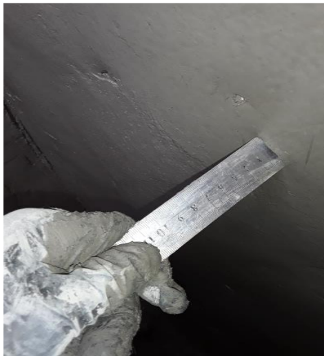
Figure 3-12. Measuring the coating thickness with a ruler
