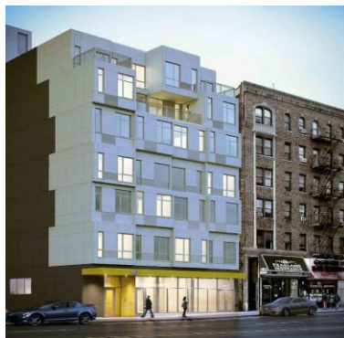
(a) 6-storey apartment, New York, USA [29]
