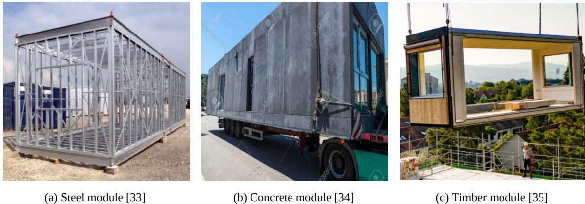
Figure 2.4: Modules in different materials
