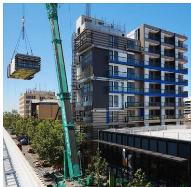
(b) 10-storey apartment, Melbourne, Australia [1]
