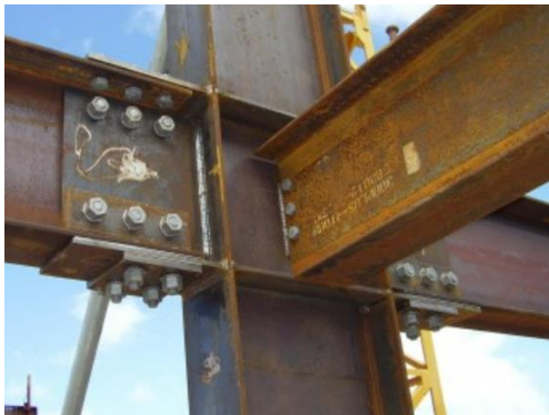
(a) Typical steel structure [51]
