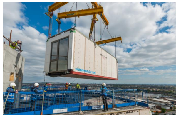
(b) Modular construction [15]
