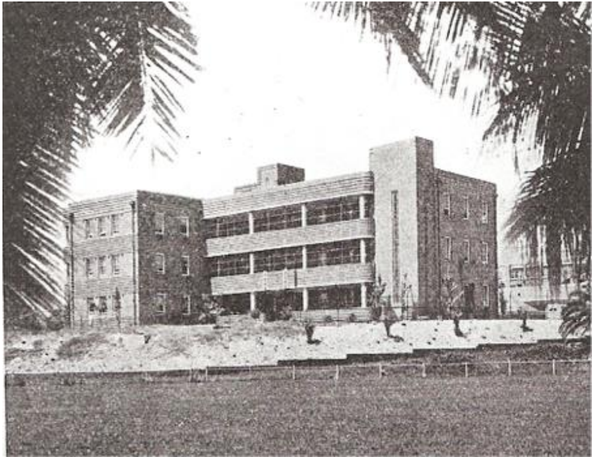
The Psychiatry and Neurosurgery Pavilion at the Royal Prince Alfred Hospital, viewed from St John's College Oval. Royal Prince Alfred Hospital Annual Report. 1938. Page 19. Courtesy: Museum and Archives, Royal Prince Alfred Hospital.
