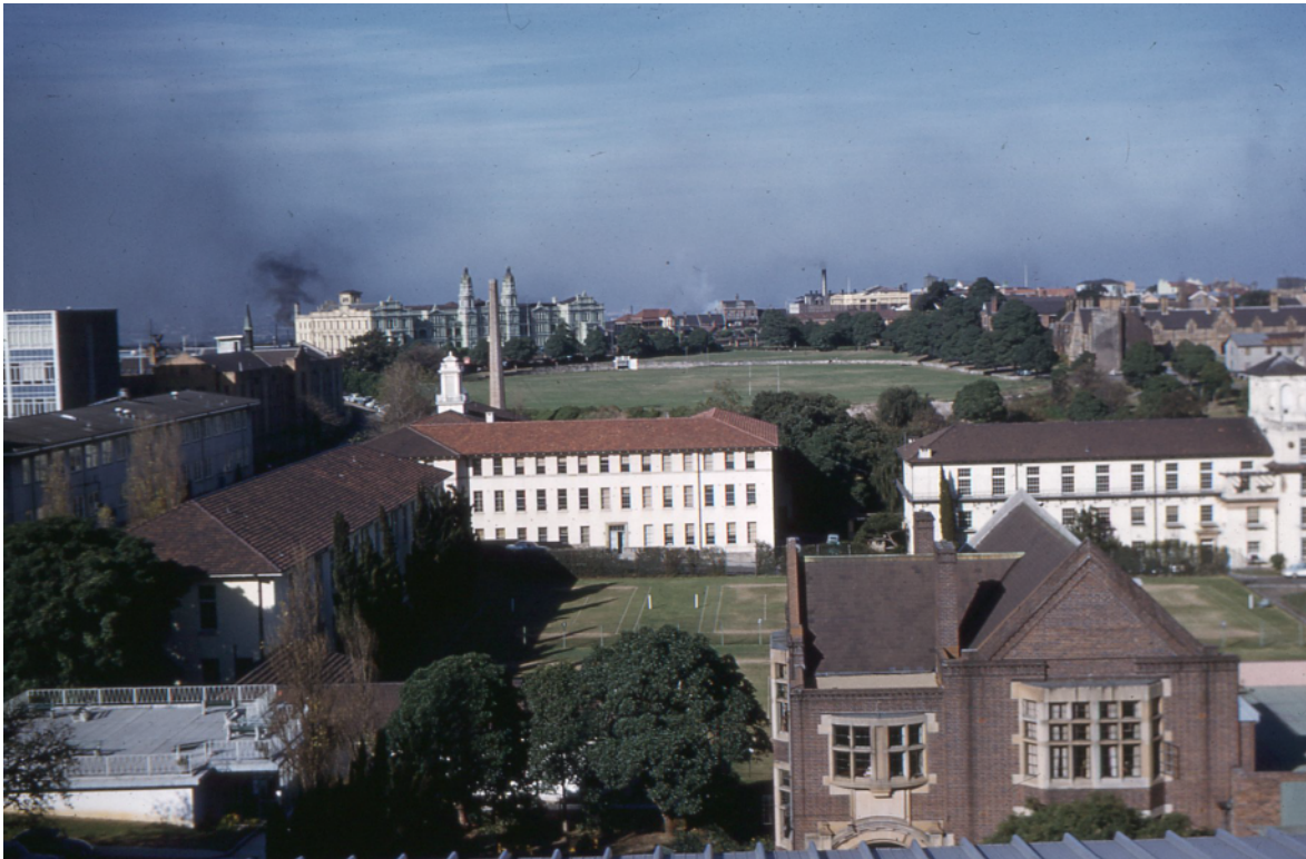
3.13 Looking south from the top of the Mungo MacCallum building 1/6/1961.
