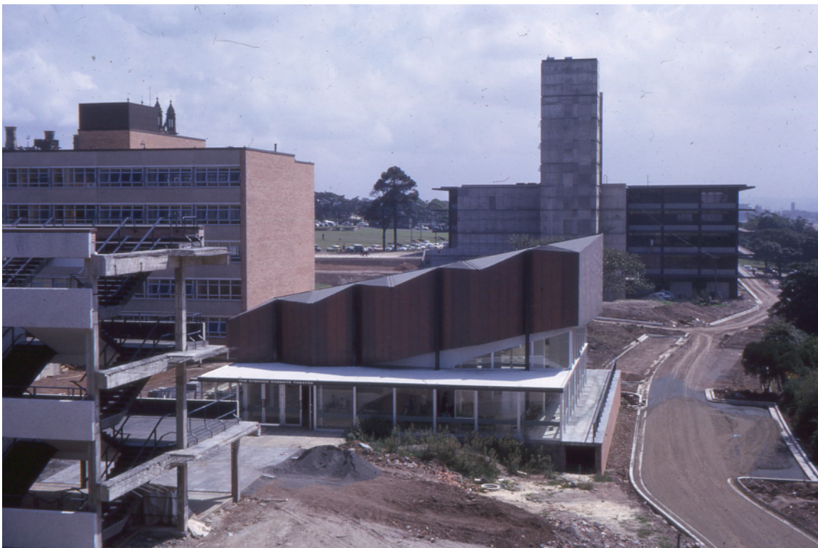
6.35 Looking east from 5th floor of Carslaw Building, 3/1963.
