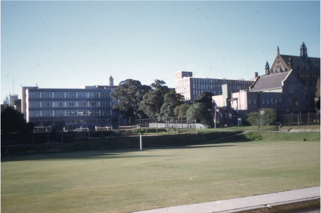
4.21 Looking north from outside the Physics building 16/6/1961.
