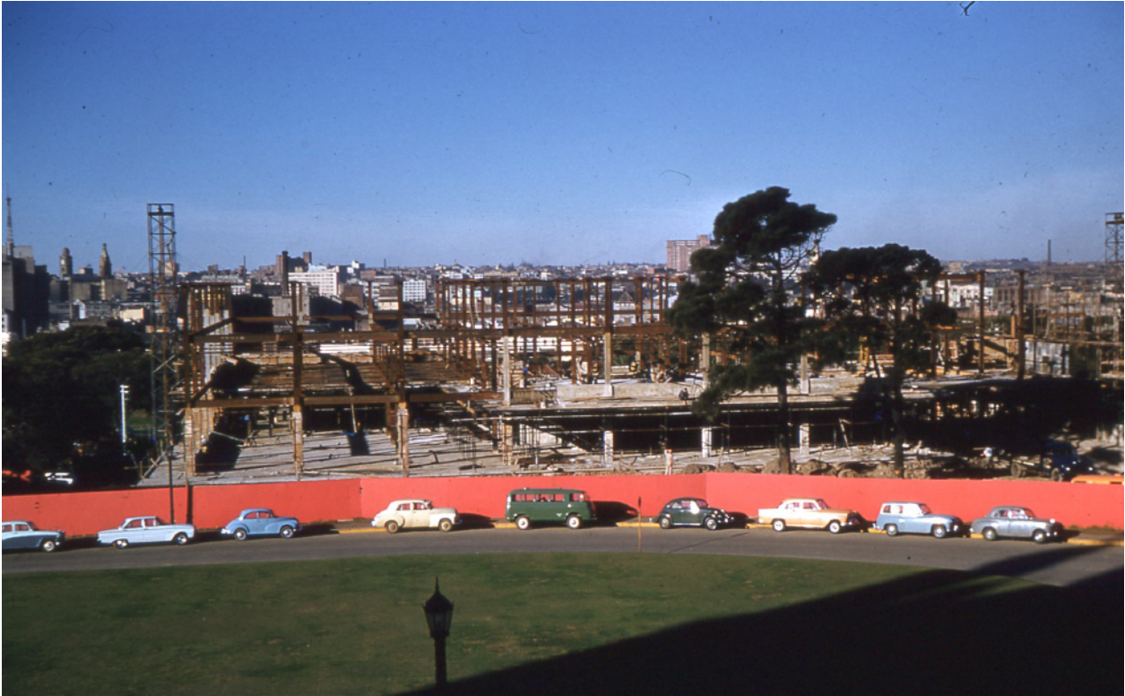
4.20 Work commencing on the new Fisher Library, 16/6/1961
