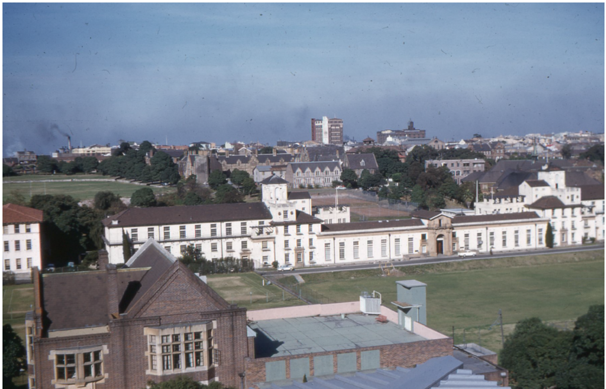
3.15 Looking south from the top of the Mungo MacCallum building 1/6/1961.
