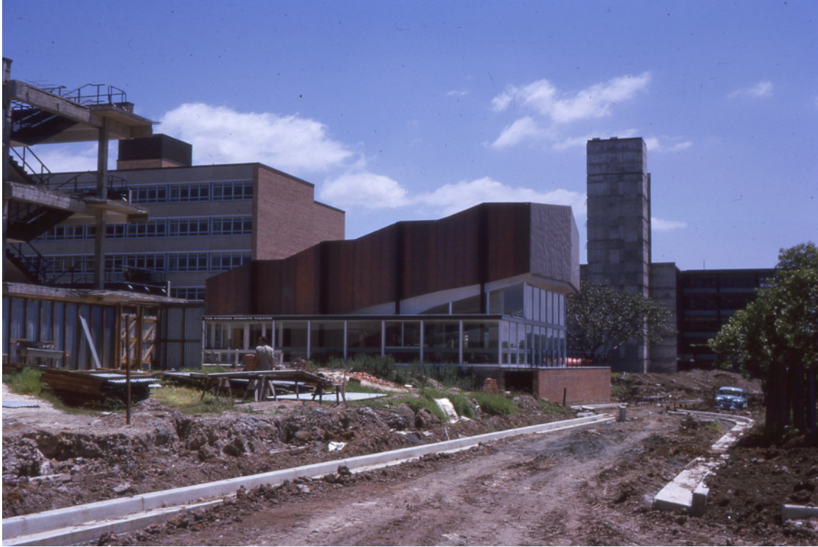
6.27 Looking east from Barff Road, adjacent to Victoria Park, 5/2/1963.
