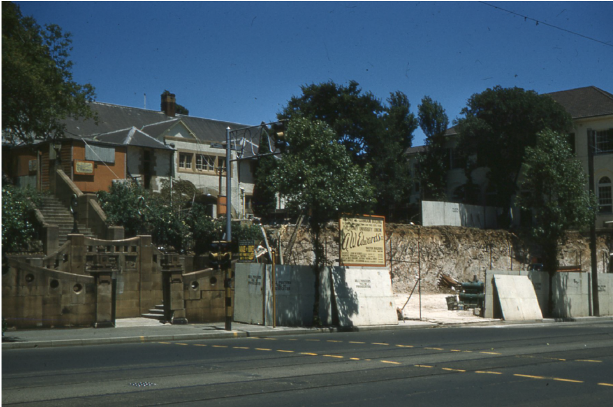
1.16 The demolition site of the old Union Theatre on Parramatta Road 26/1/1960
