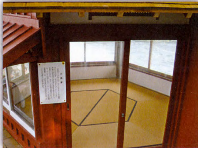
Okakura’s Sea Side Small Summer House, Photograph Kedar Vishwanathan 2008.
