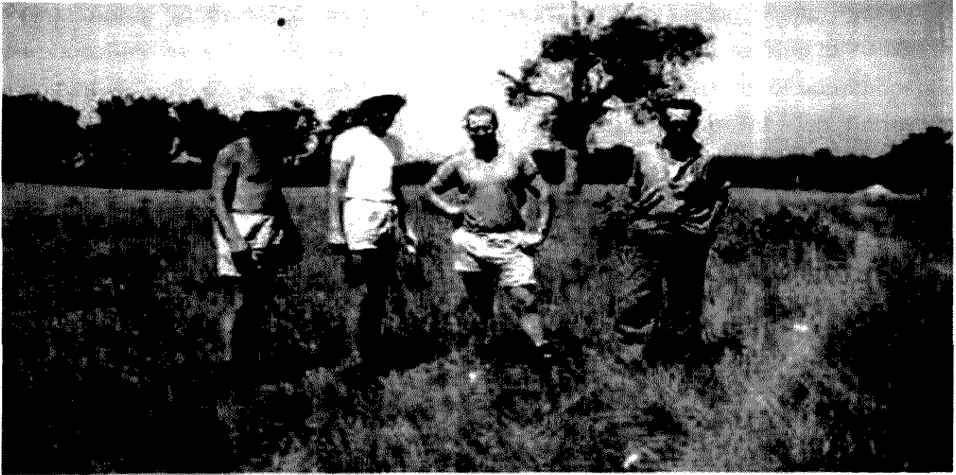
Figure 4.17 Construction workers at Tocal before commencing building of the college, February (?) 1964 (from the Tocal website ( http://www.tocal.com )).
