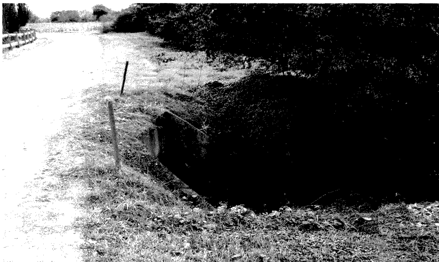
Figure 2.7 Modern flood-level drainage outlet of the northern end of Tocal Homestead Lagoon via a concrete culvert, running beneath the main access road to the Tocal Homestead, 1998.
