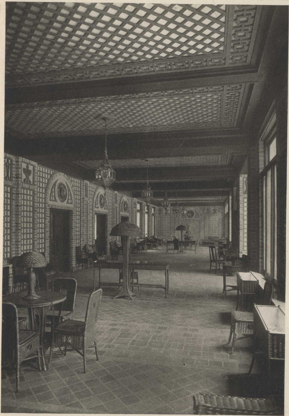
ENTRANCE LOGGIA, FACING 16TH STREET.
