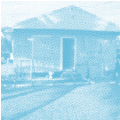
Timber and steel framed demountable housing.
