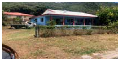
The exist house
