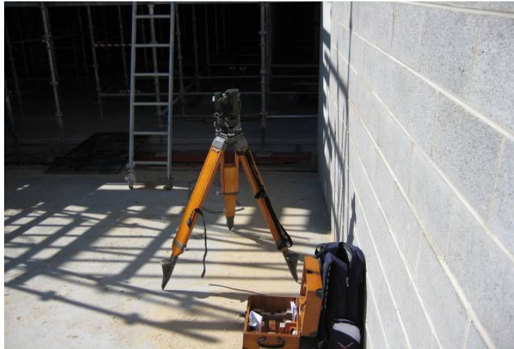
Figure 4: Theodolite employed for storey out-of-plumb measurement
