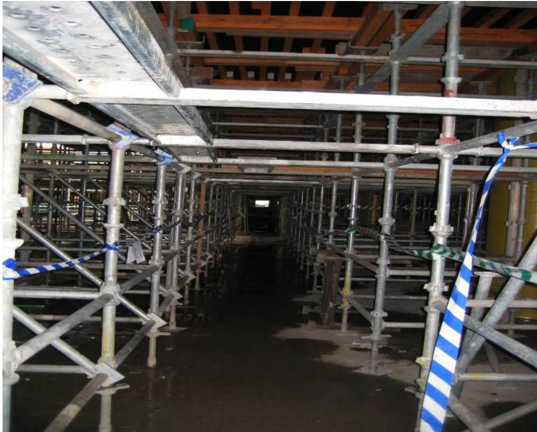
Figure 1: Cuplok scaffold systems
