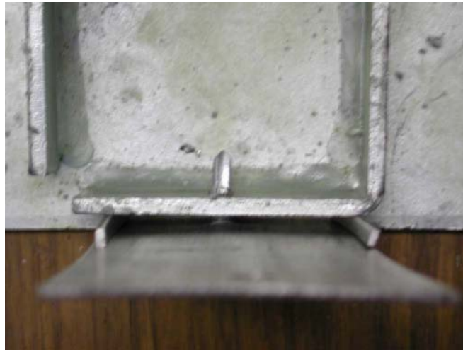
Figure 4: Packing replaced by edge packing
