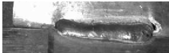
Fig. 17 HAZ failure at the tension end of a flare-vee weld in 1.5-mm sheet steel
