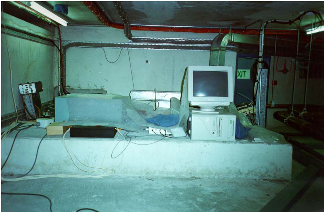
Fig. 2 Accelerometers, signal conditioning and data logging equipment, Brisbane Airport Control Tower
