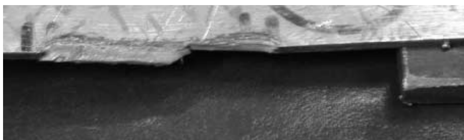
Fig. 8 Weld failure of double-lap longitudinal fillet welded connection in 3.0-mm sheet steel
