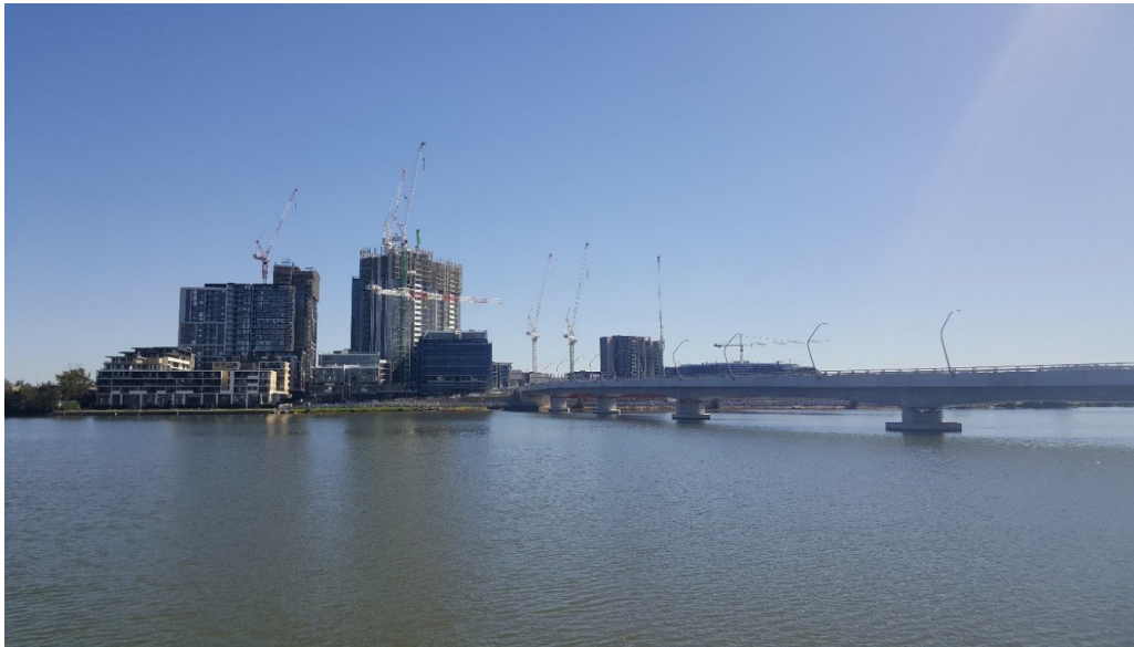
Public transport bridge from Wentworth Point to Rhodes, provided under a VPA (Credit: Laura Crommelin)
