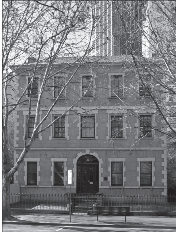
Figure 3: 300 Queen Street, Melbourne (Source: Peter Maltezos).
