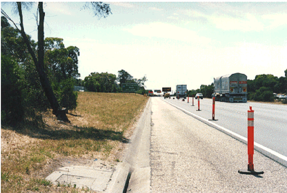
Figure 6: Traffic Management in the Work Zone
