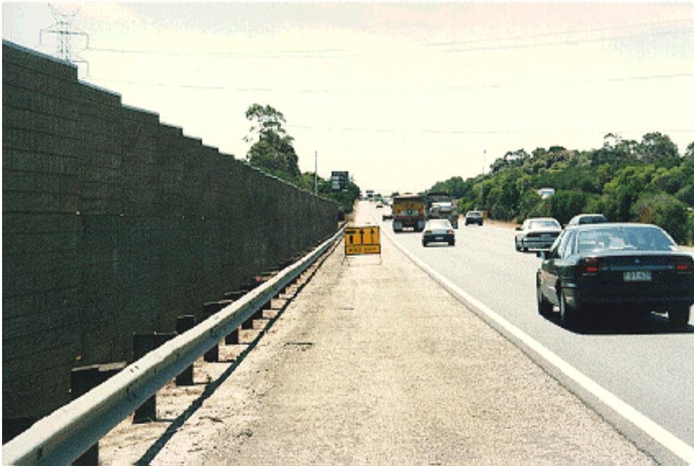
Figure 5: Static Signs in the Works Zone
