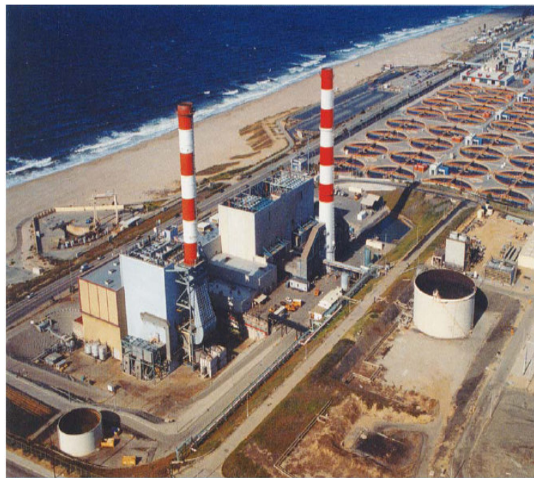
Figure A.6 Shows Encina Desalination plant is located on the site of the Scattergood Generating Station at the southern Coast of California.
