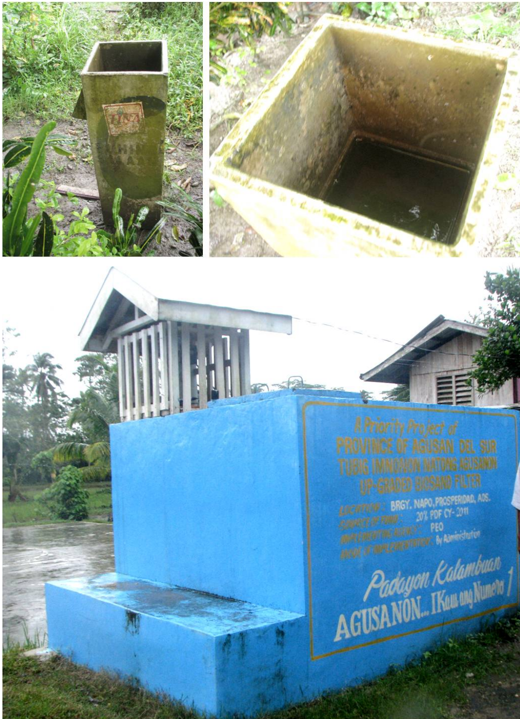
Top photos: Show the abandoned state of the household biosand filters distributed to the Napo households; Bottom: The 'improved' Biosand filter that was designed by WATSAN Centre Source: Photographed by author, Napo, 2013.
