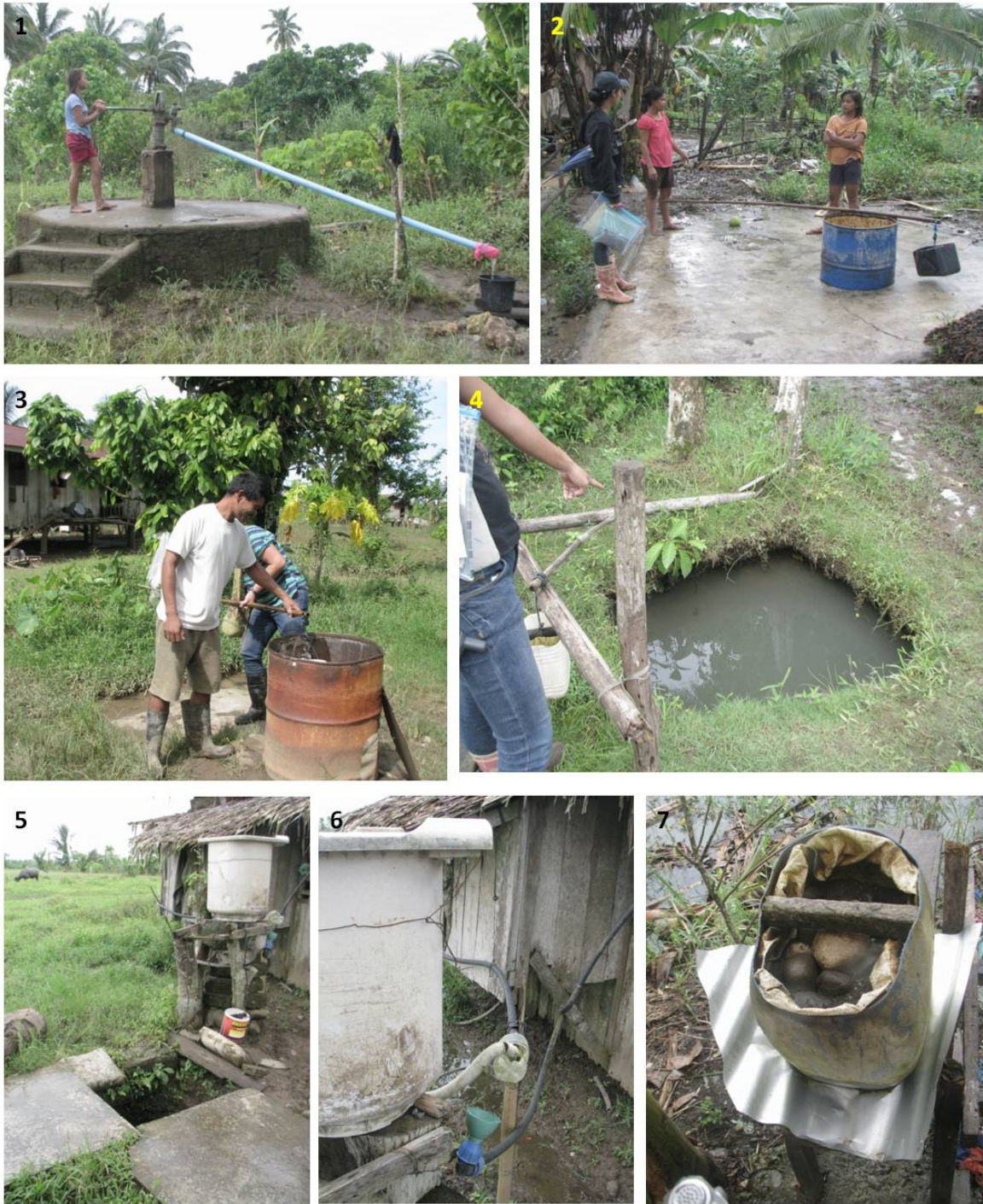
Photo 1: Privately owned water hand pump used for drinking; Photo 2: Dug well with a cemented apron around the well and a barrel covering the hole head; Photo 3: Hole head with barrel. Photo 4: Dug well; Photo 5-6: Improved home water system with filter - a barrel containing sediment and charcoal to filter the water placed beside the well so collected water is poured into the barrel and a pipe channels water straight to the house's kitchen. Photo 6: Another household filtering device
