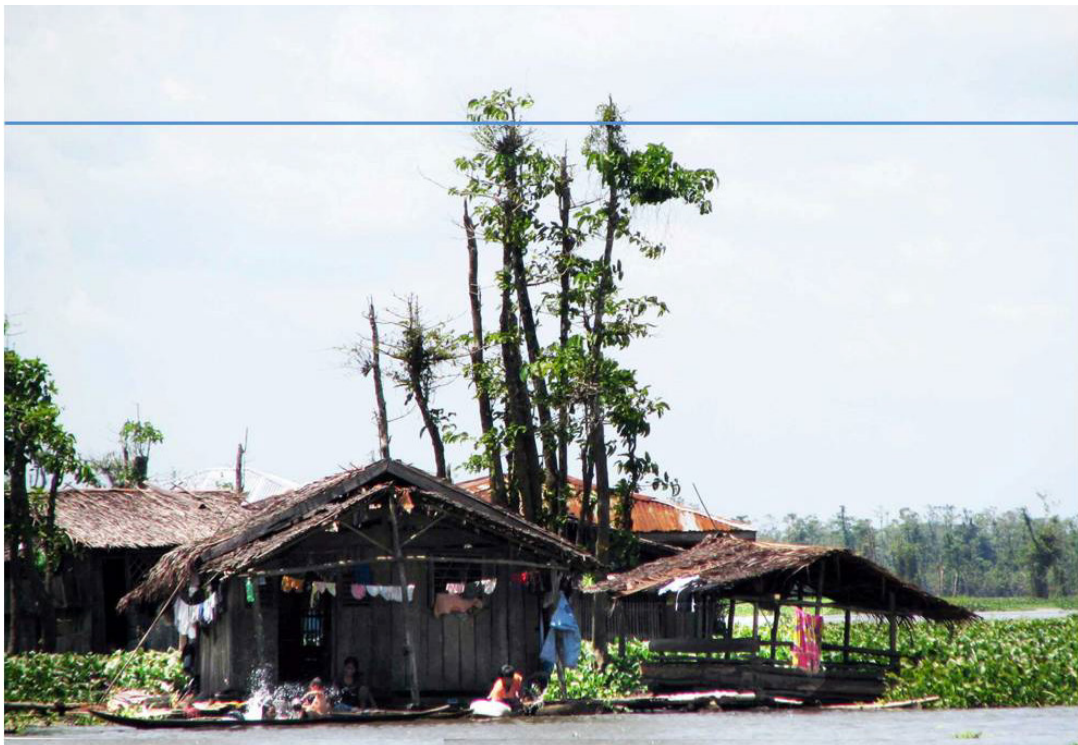
Figure 7.1: Floating houses in Panlabuhan (noting the water level)
