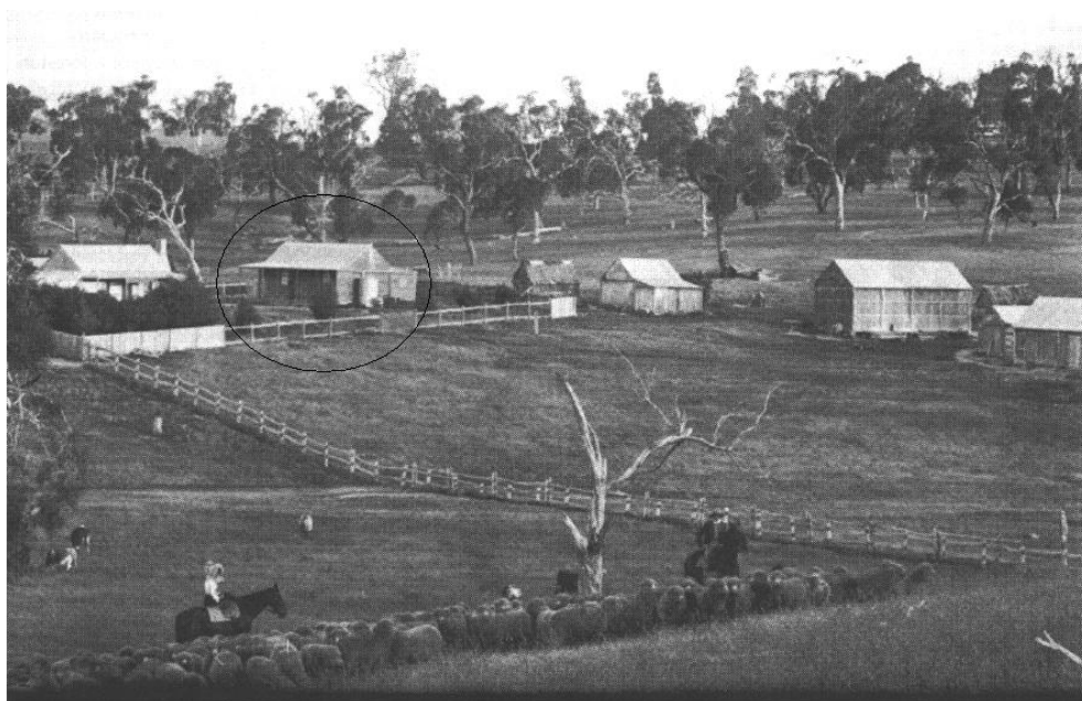
Image 18. The Wong family store at Crookwell, c. 1909. The circled building is the store and the family's home is the building to its left. Photograph by Henry Wong, Powerhouse Museum Collection
