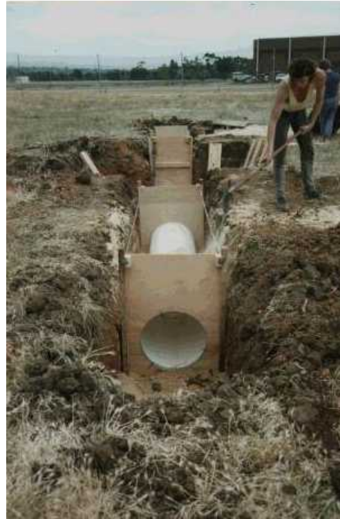
Fig 4-4b. Pipe in position ready for backfilling
