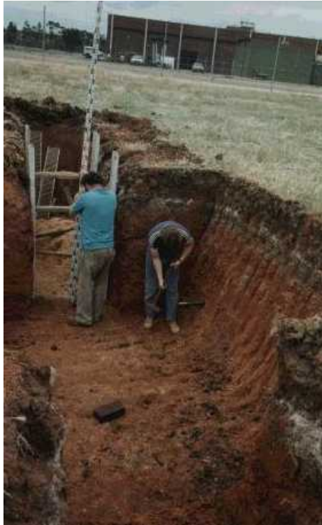
Fig 4-4a. Excavation and sampling of the natural soil
