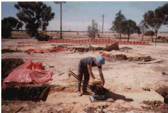
Fig 4-4c. Compaction of backfill with vibrating plate compactor
